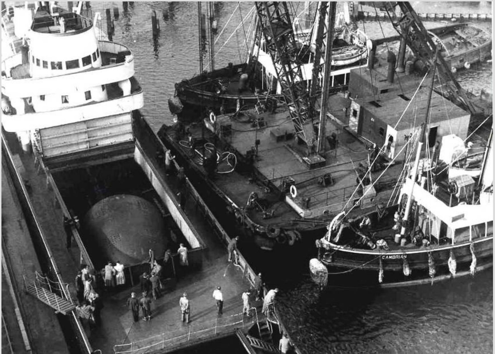
Floating crane ready to lift the Bessemer converter
