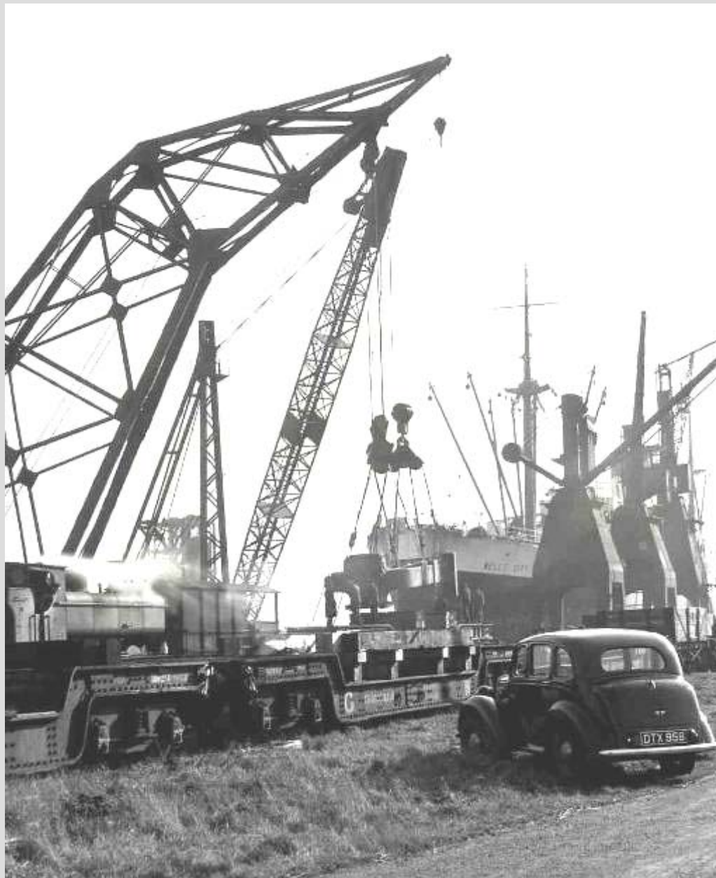
Piece of housing machinery being discharged
