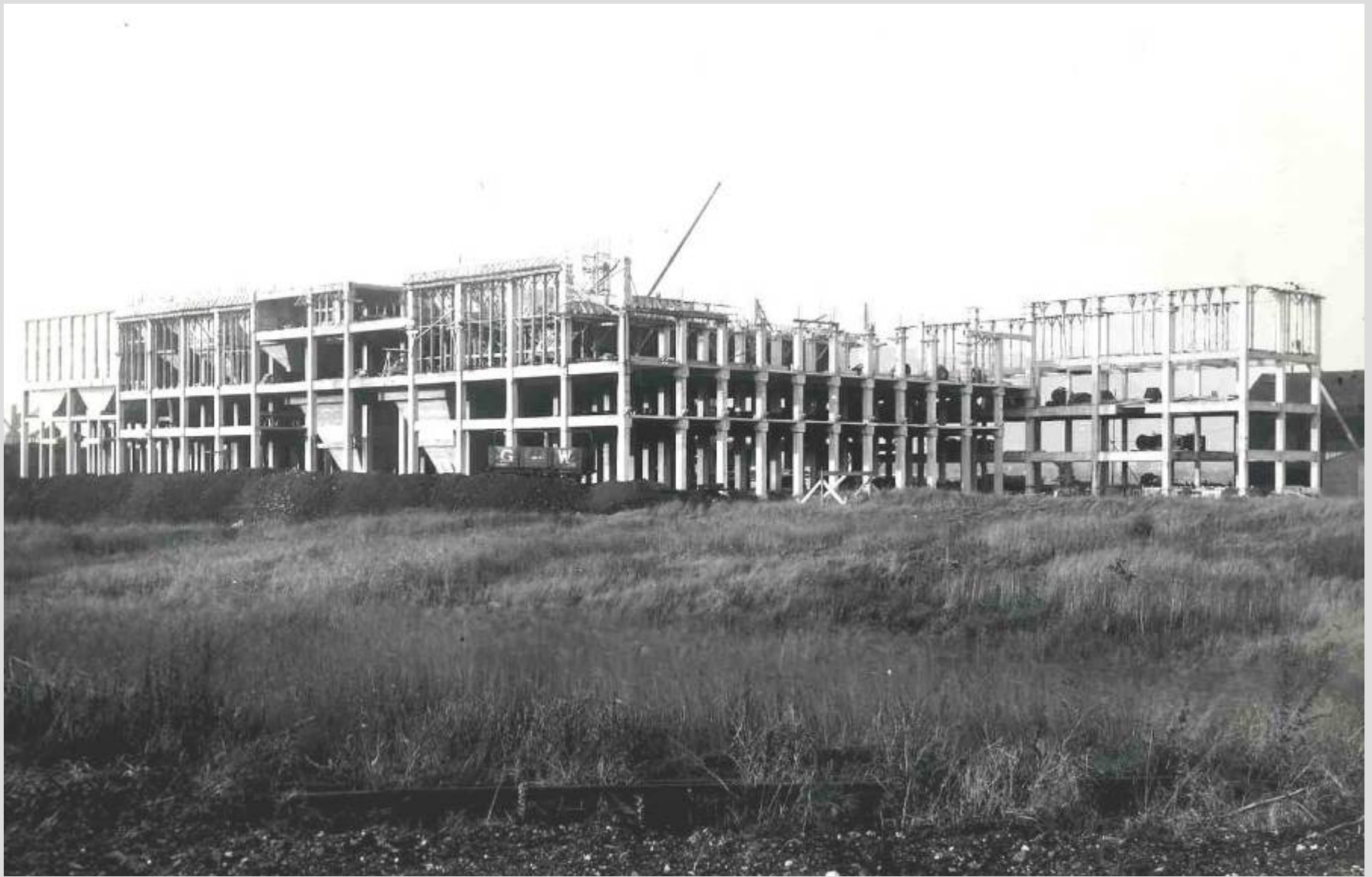
Phoenix fuel works under construction
