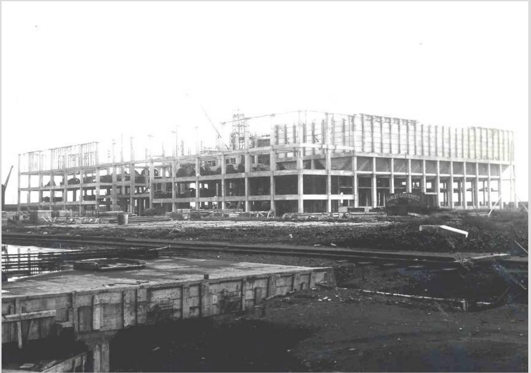
Phoenix fuel works under construction
