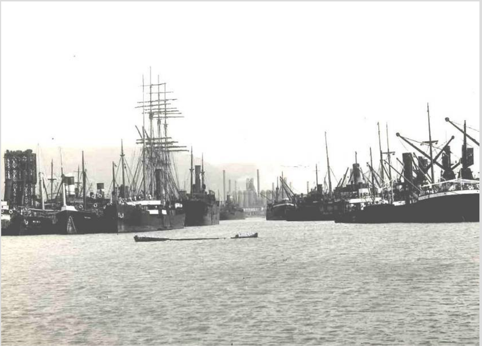
View of Port Talbot Docks
