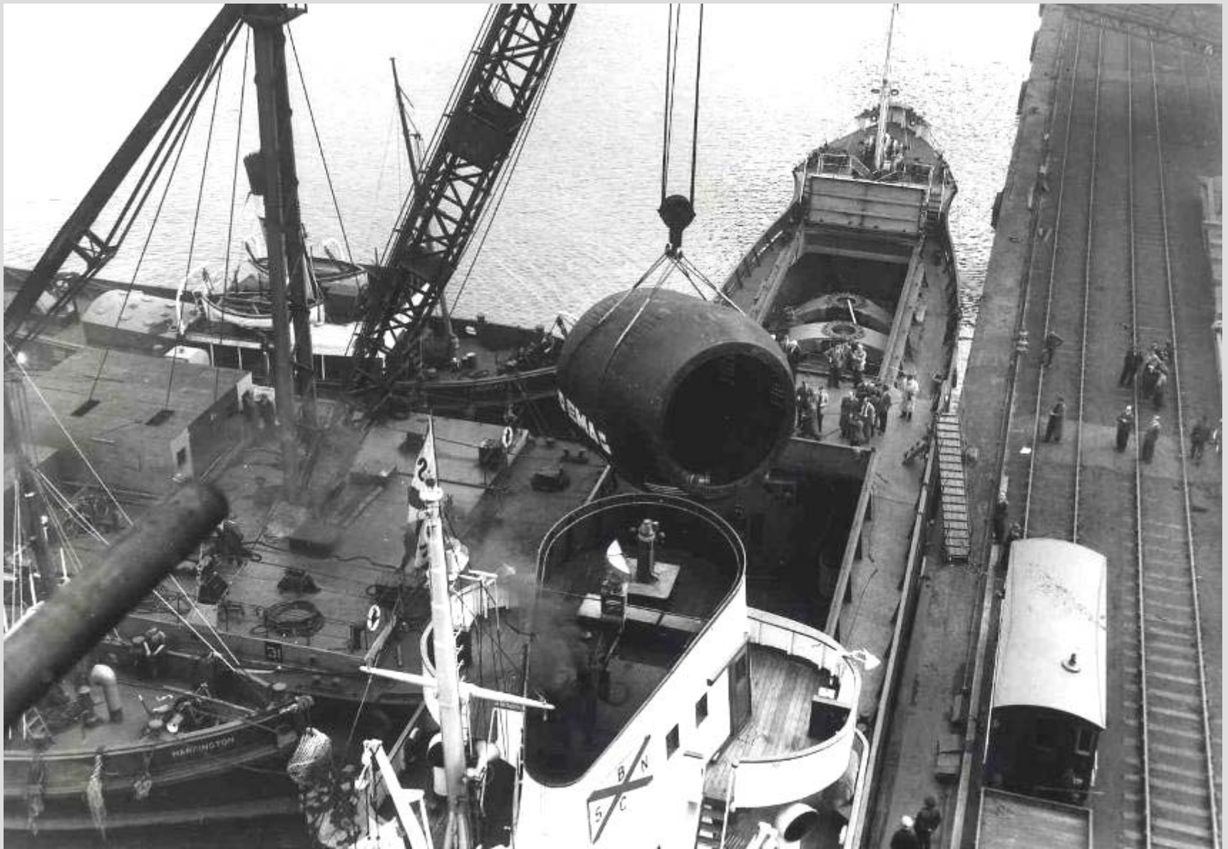
Discharge of a 50 ton capacity Bessemer Converter
