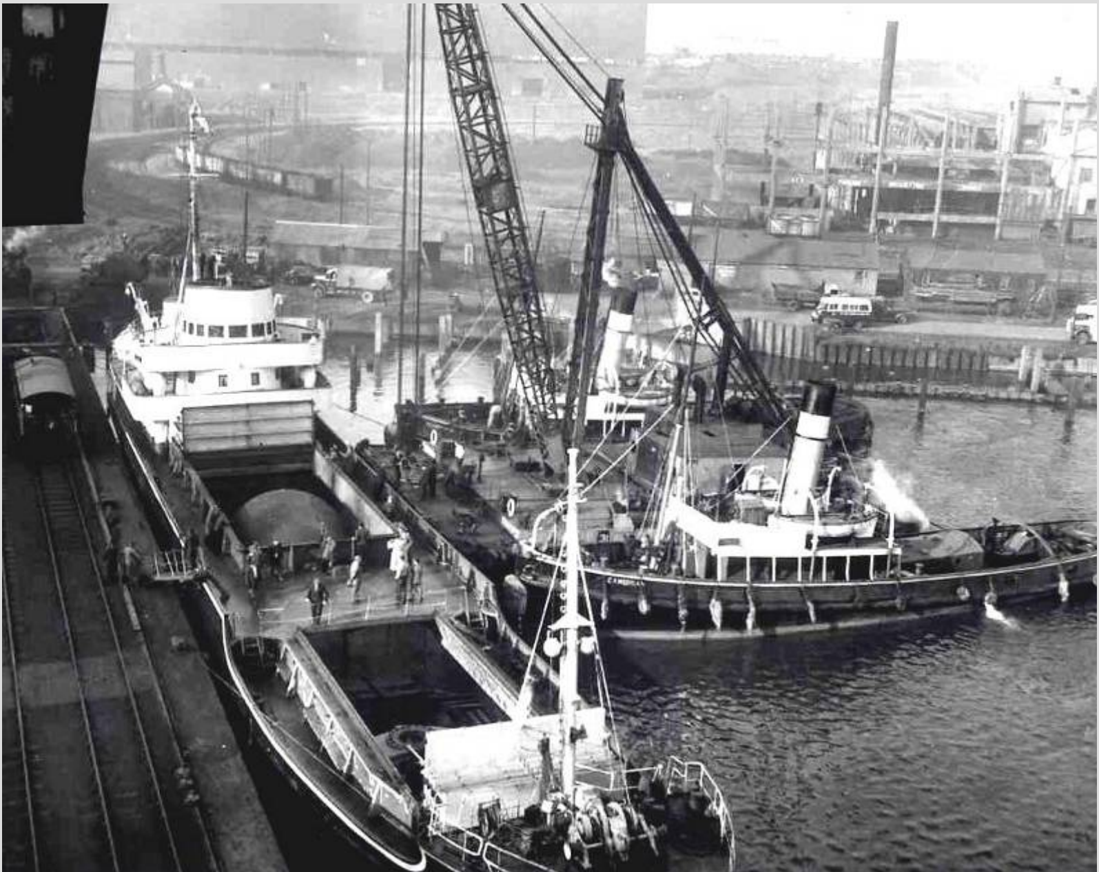
Discharge of 50 ton capacity Bessemer converter
