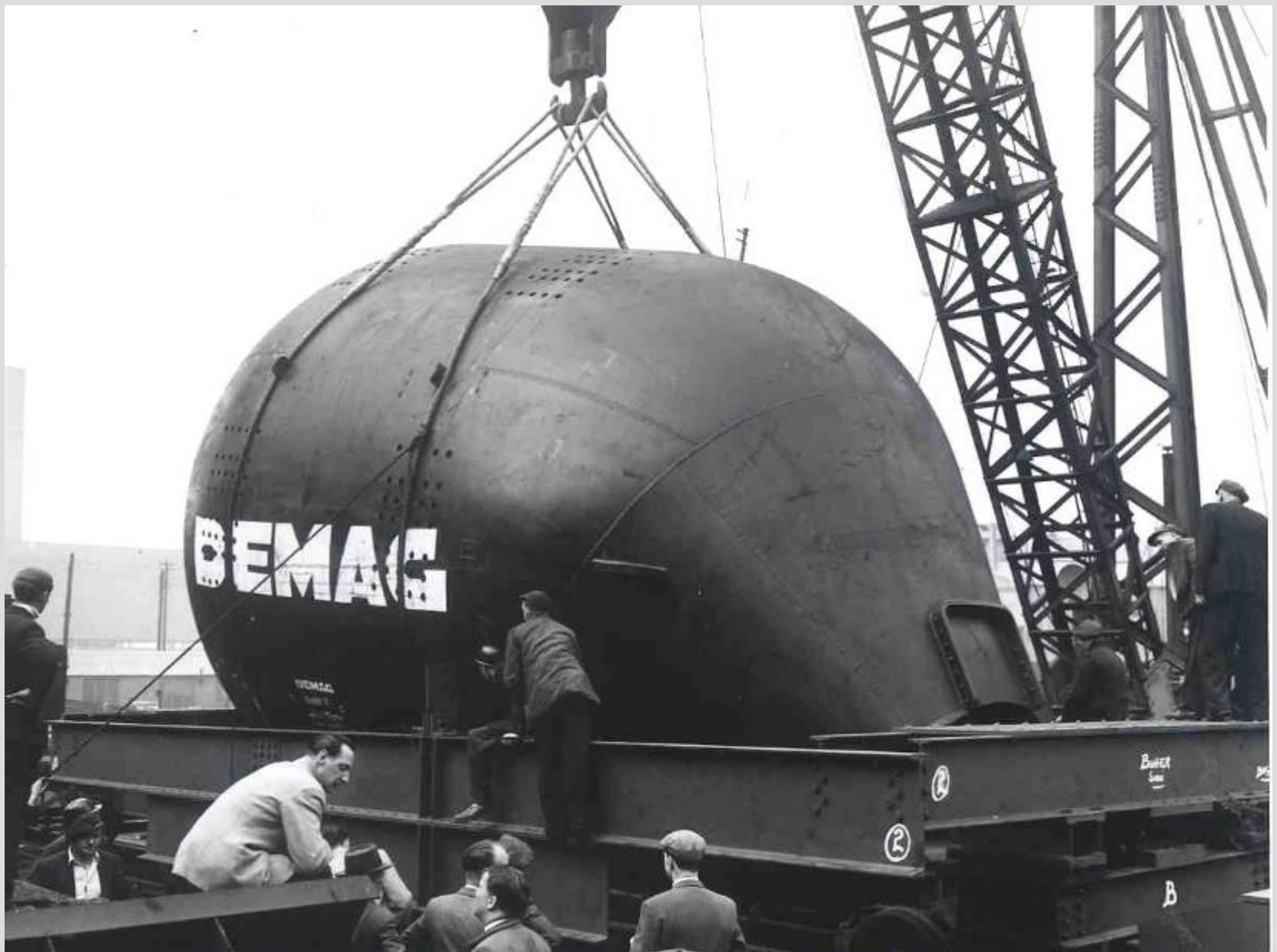
Discharge of 50 ton capacity Bessemen converter
