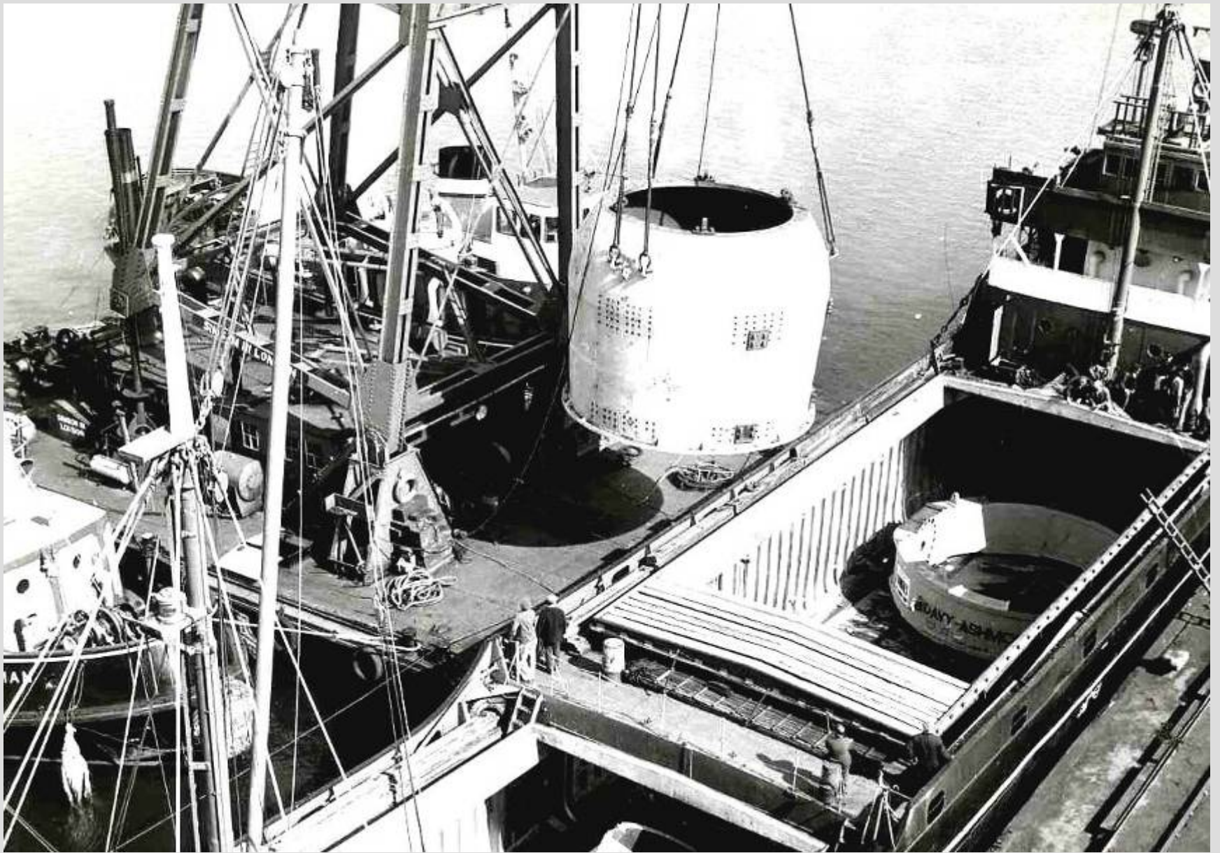
Discharge of steel converter for the Steel Company of Wales
