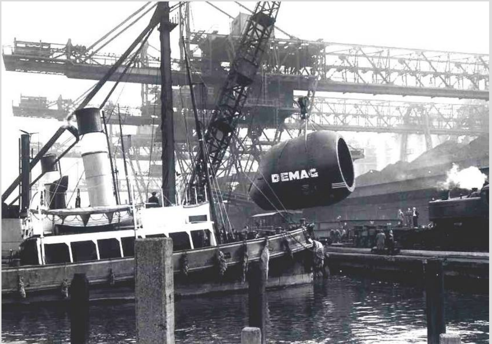
Discharge of a 50 ton capacity Bessemer Converter
