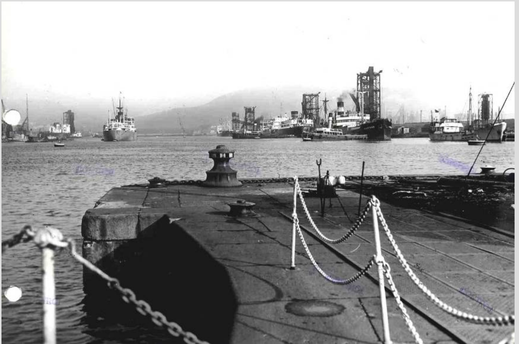
Taken from South end of entrance lock
