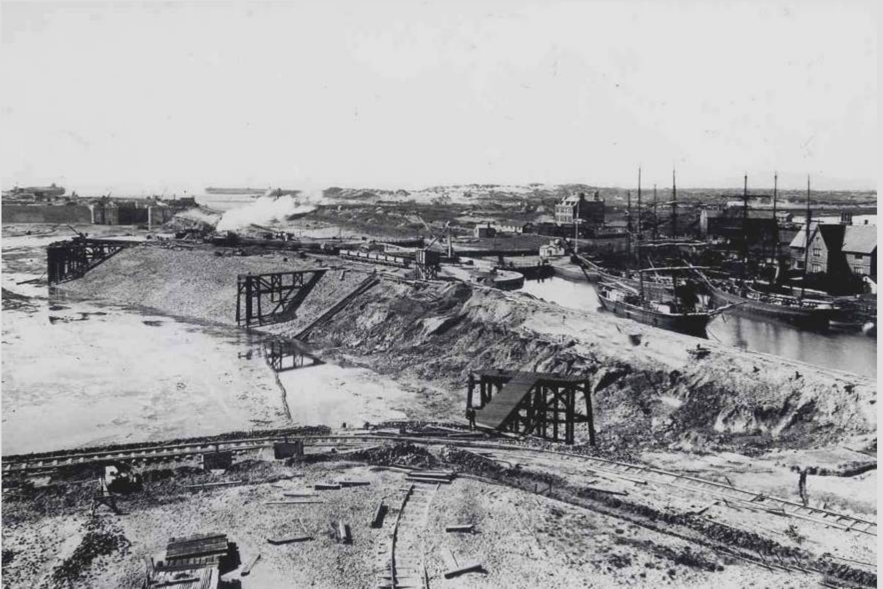
Construction of new dock, showing old lock on the right
