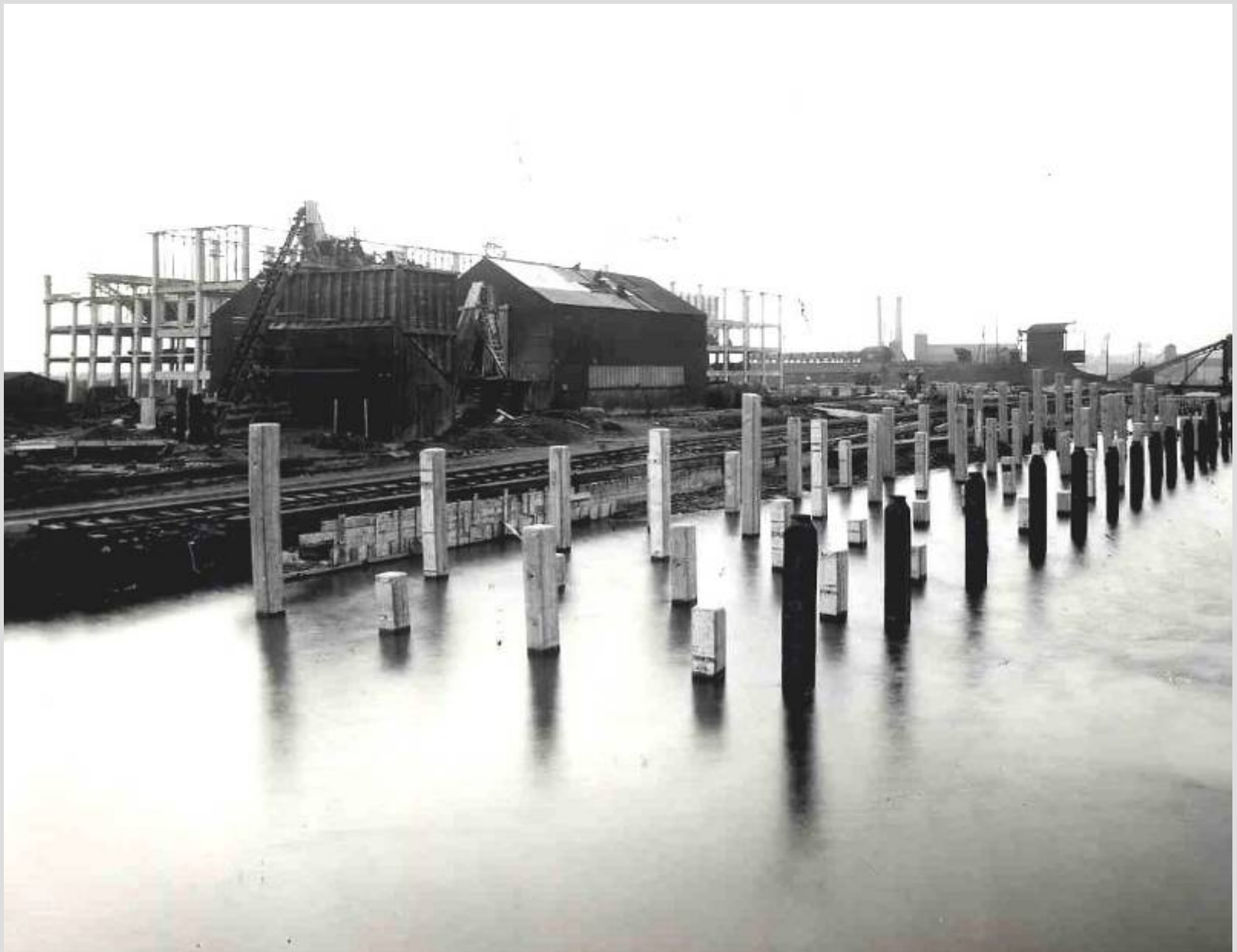
Construction of Phoenix Wharf
