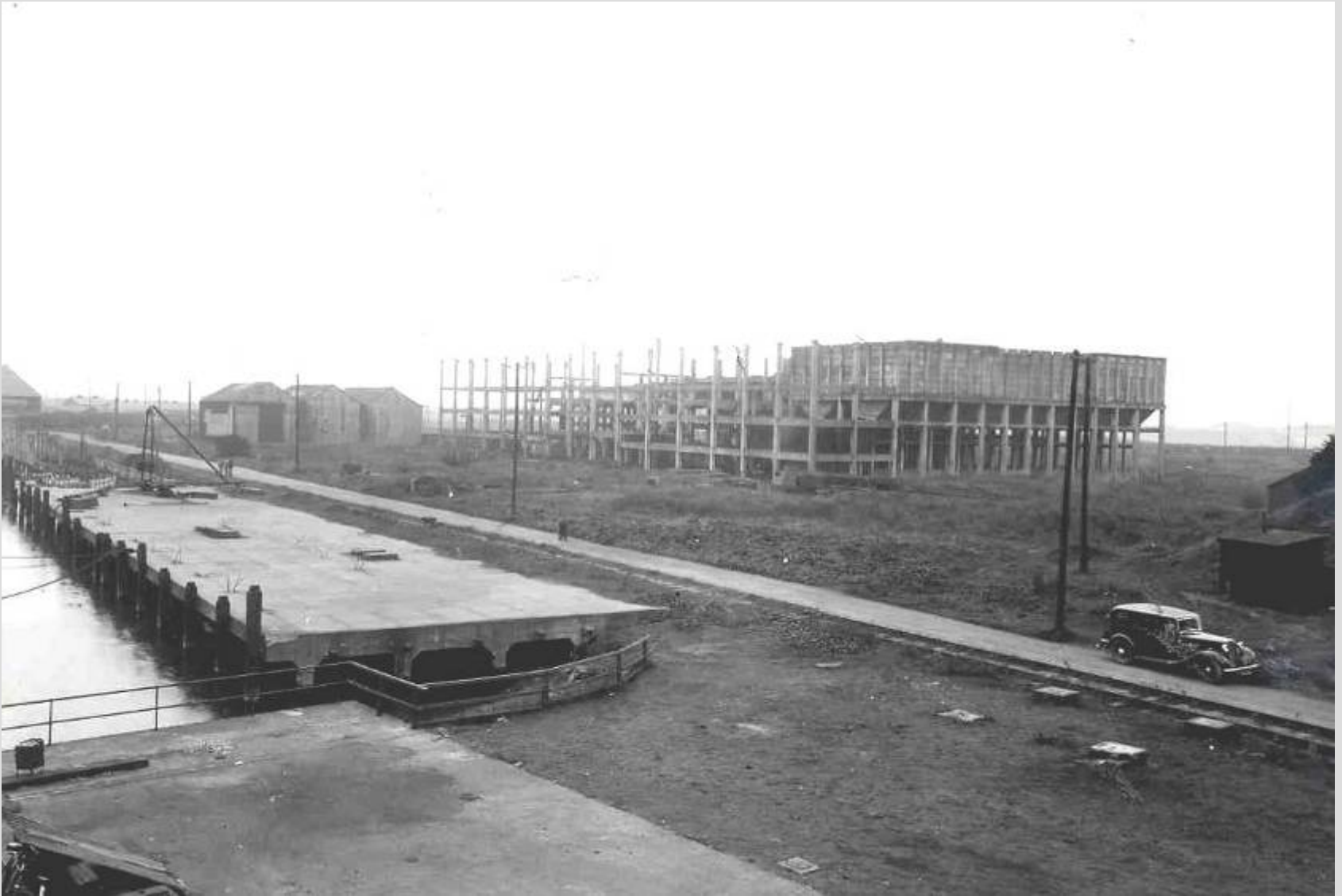
Construction of Phoenix Wharf
