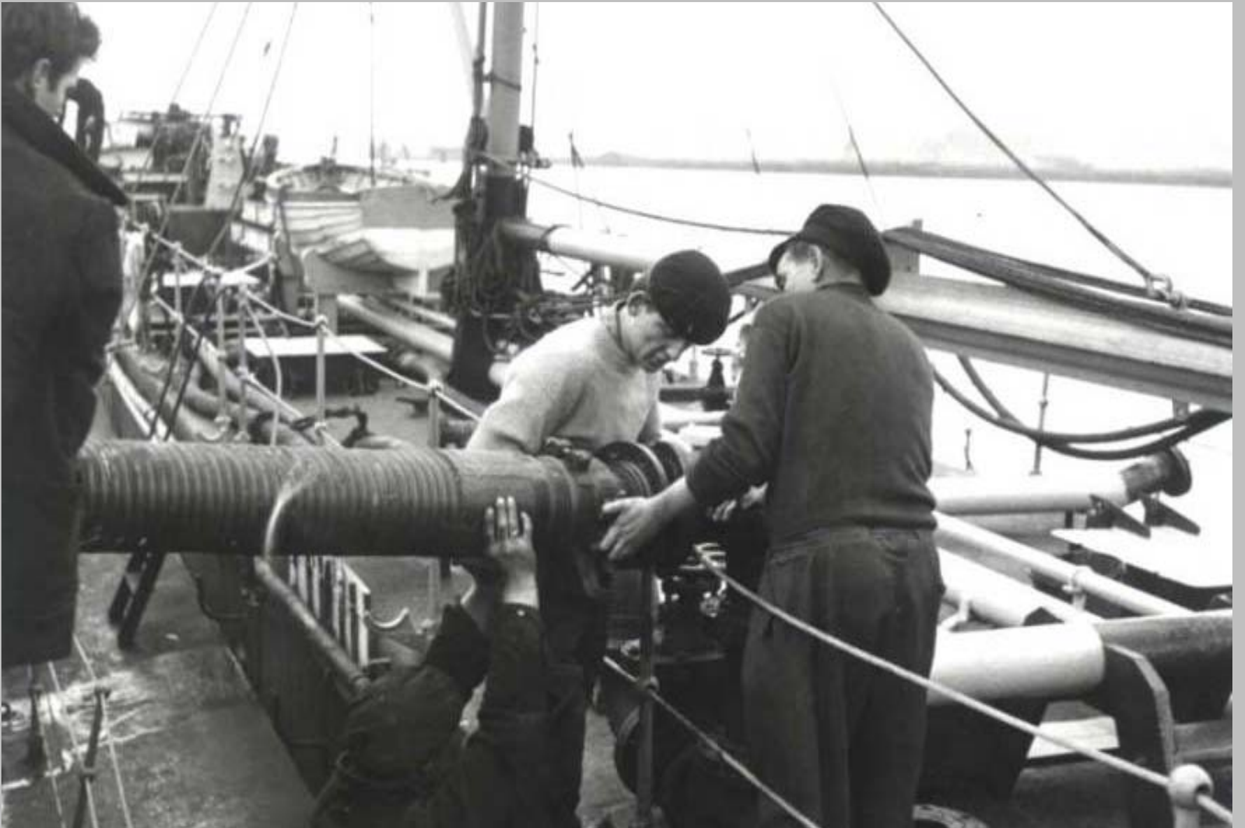
Discharging oil at Phoenix Wharf
