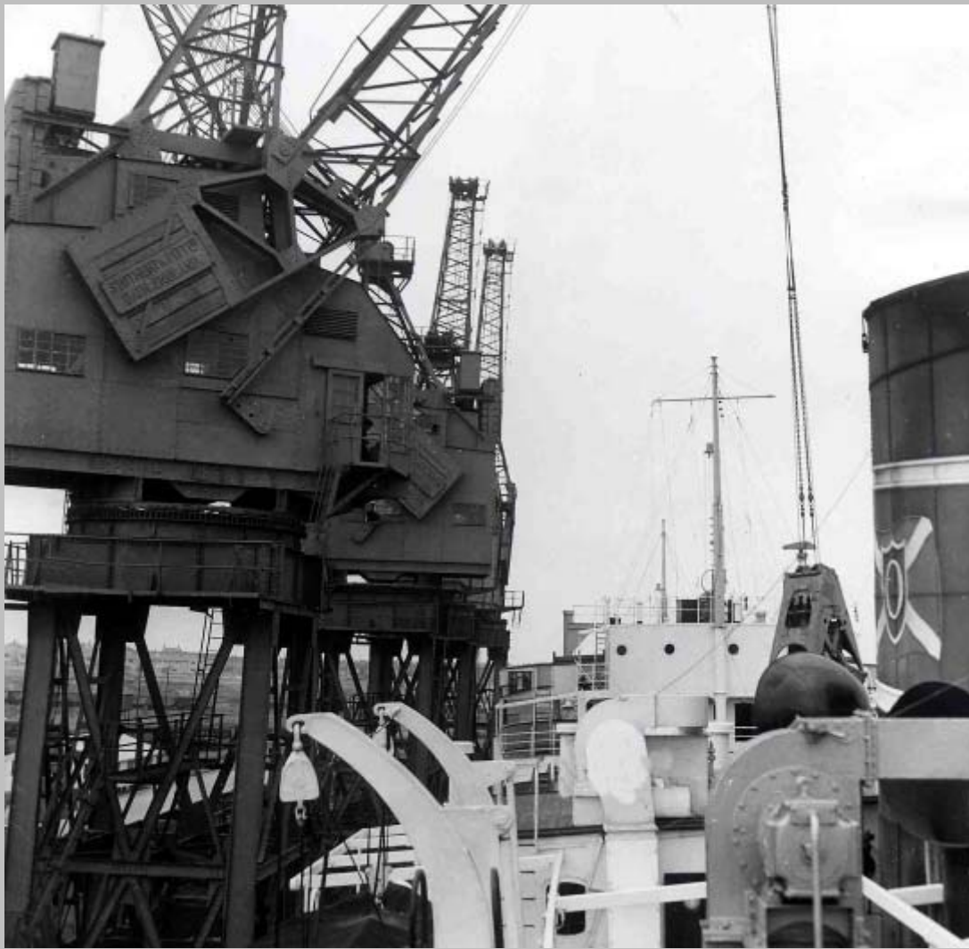
The M.V. "Ormsary" discharging 8509 tons of iron concentrates by grabs, at the new 10-ton electric crane berth , Talbot Wharf extension, Port Talbot Docks. 9th-12th August, 1959. This was the first vessel to be discharged by grabs at the berth.
