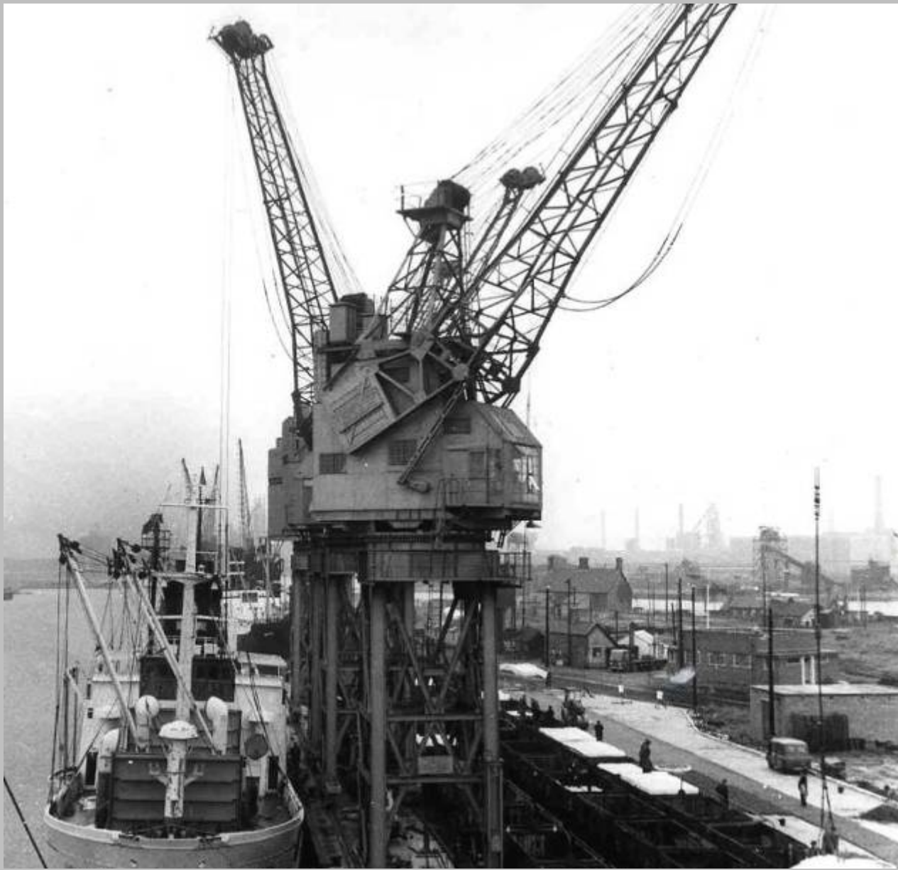
The first vessel to be dealt with at the new 10-ton electric crane berth. "Linda Dan"
