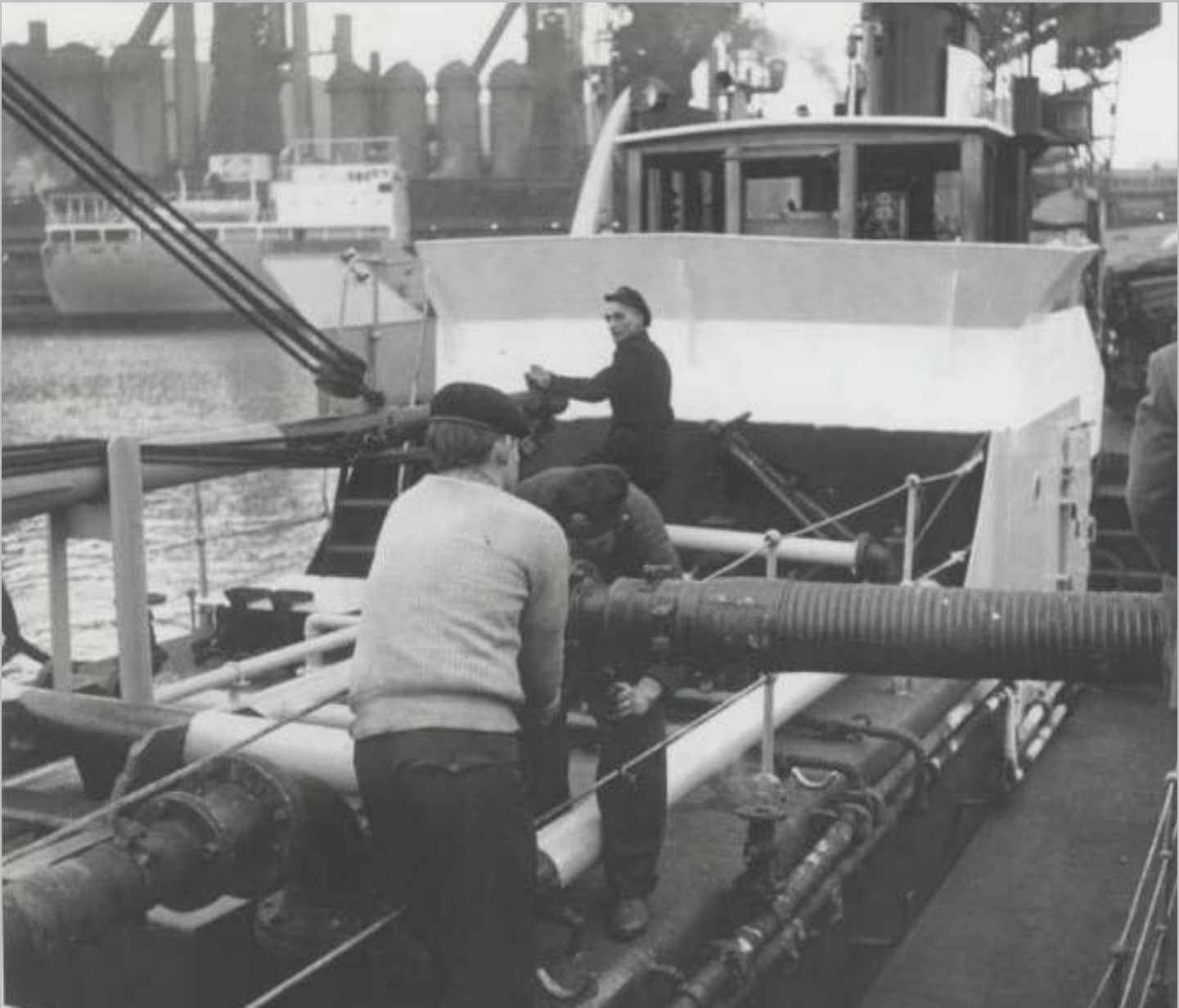
Discharging oil at Phoenix Wharf
