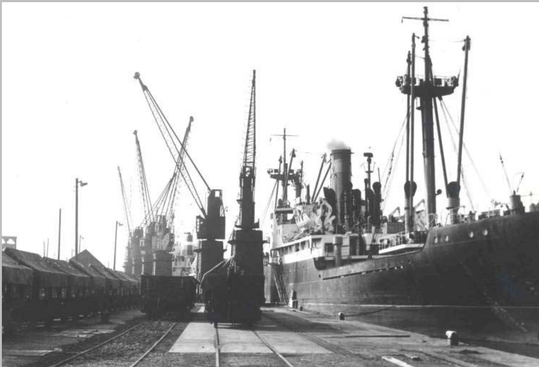
Sheeted wagons containing bundles of steel sheets berthed at Talbot Wharf awaiting shipment into Russian vessel
