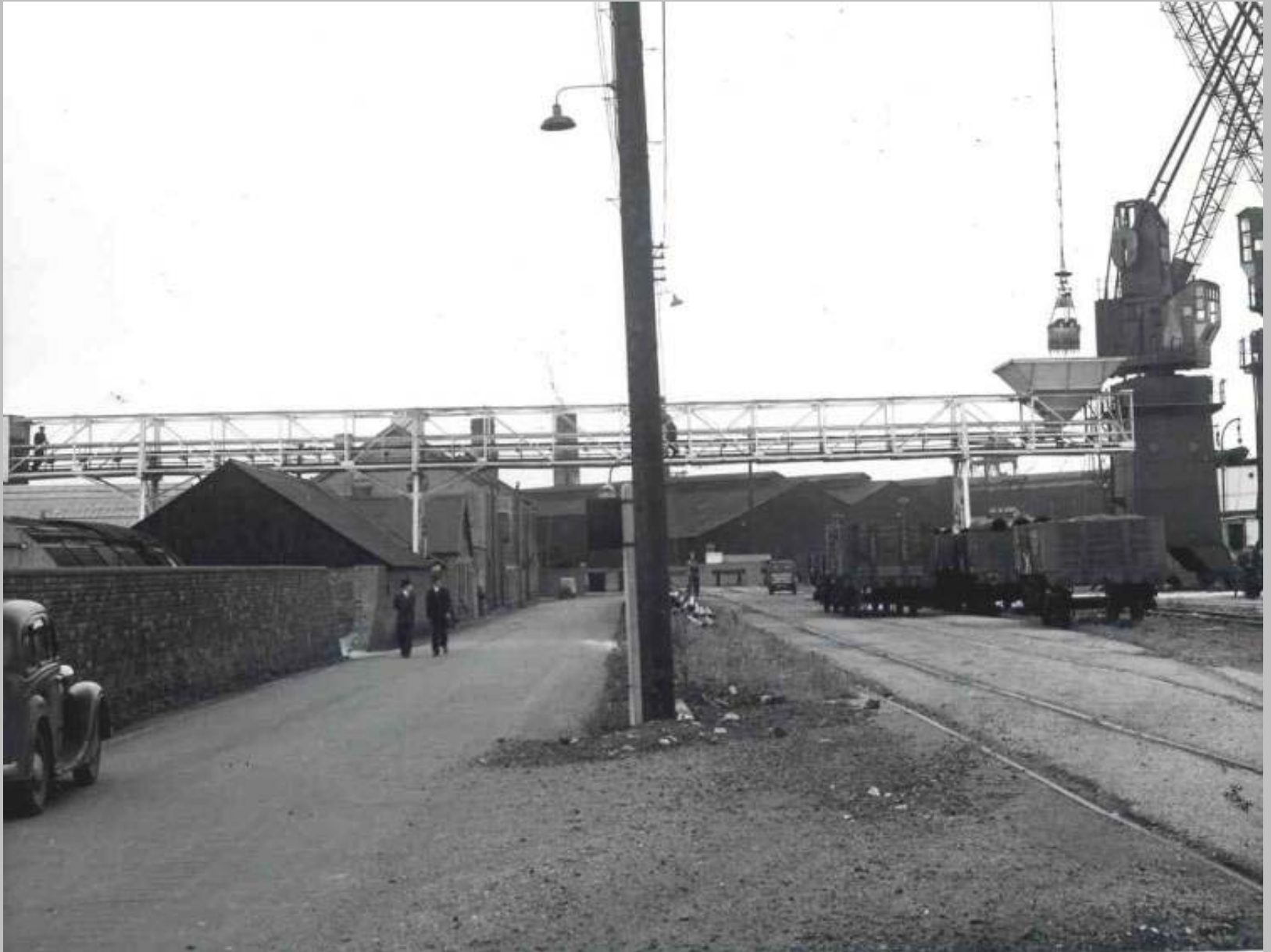
Overhead gantry with hopper and conveyor belt for carrying gypsum rock
