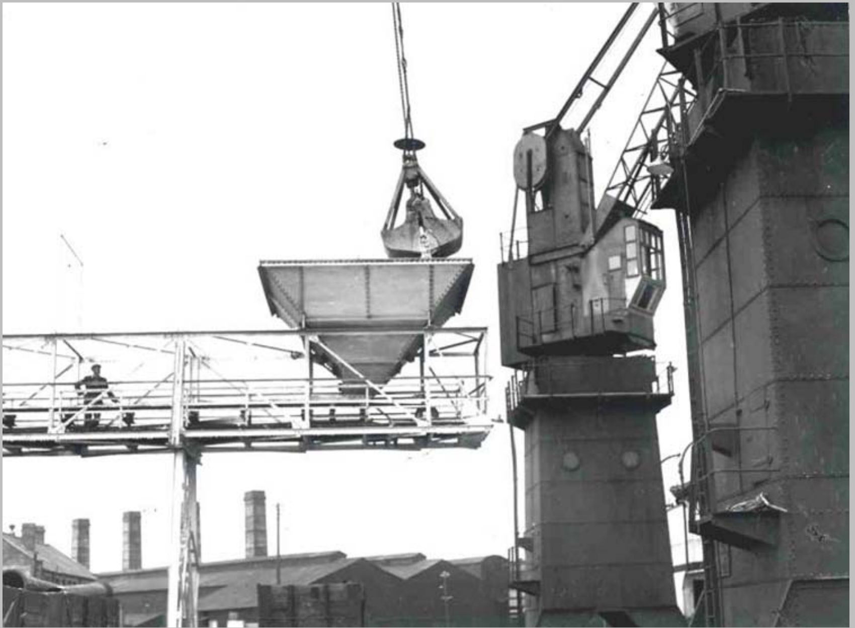
Gypsum Rock ex-ship being fed on to overhead conveyor belt through hopper
