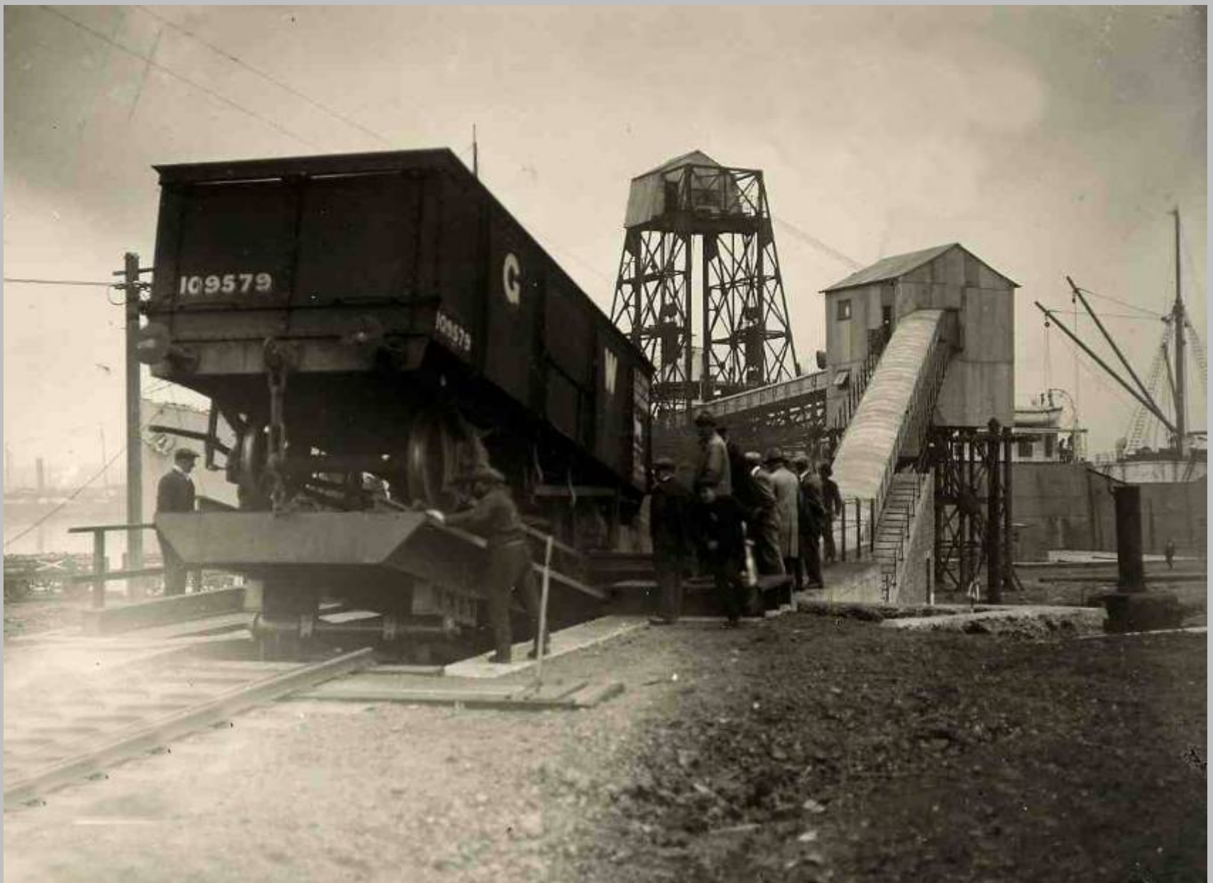
Tipping the first 20 ton wagon at No. 10 conveyor
