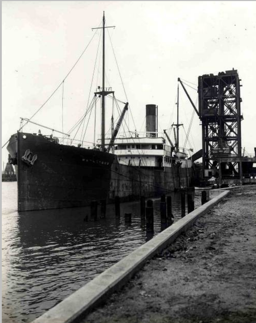
ss 'Maplewood' loading coal in 1928
