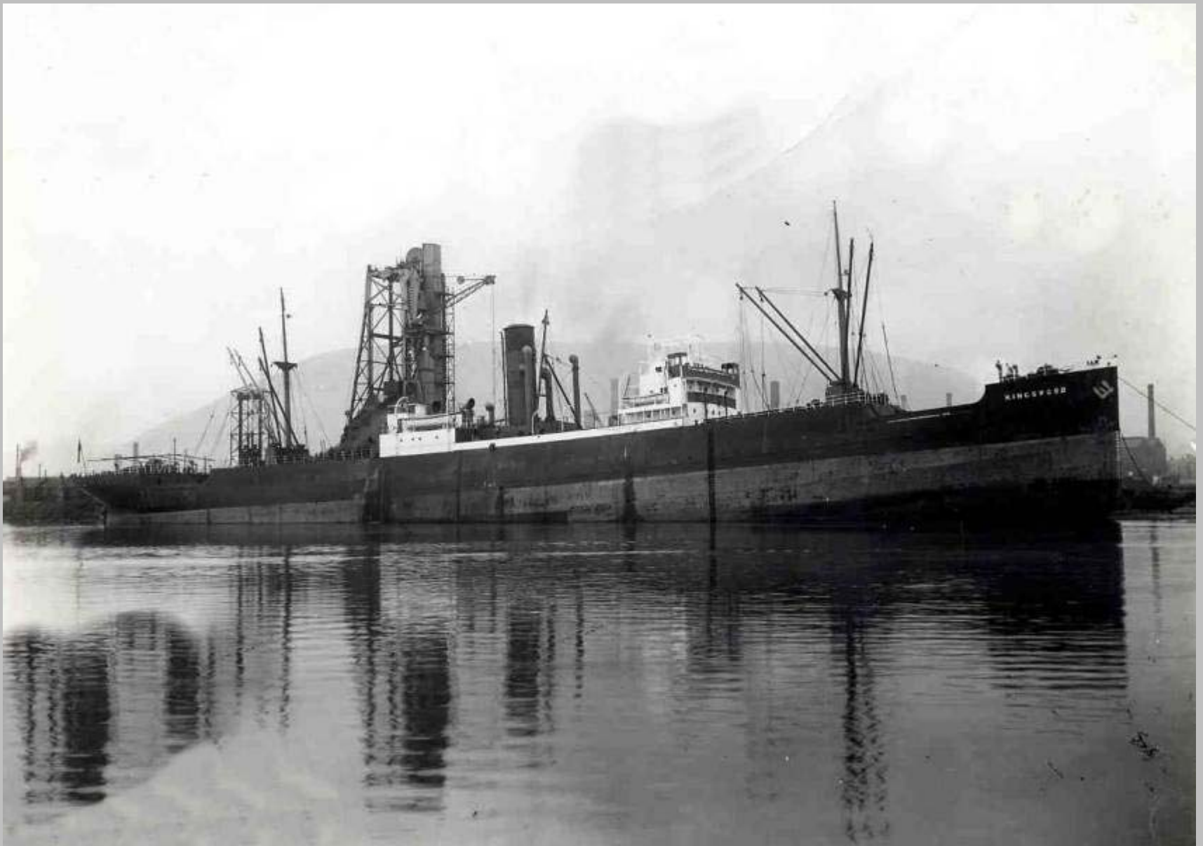
ss 'Kingswood' on new 20 ton coal hoist
