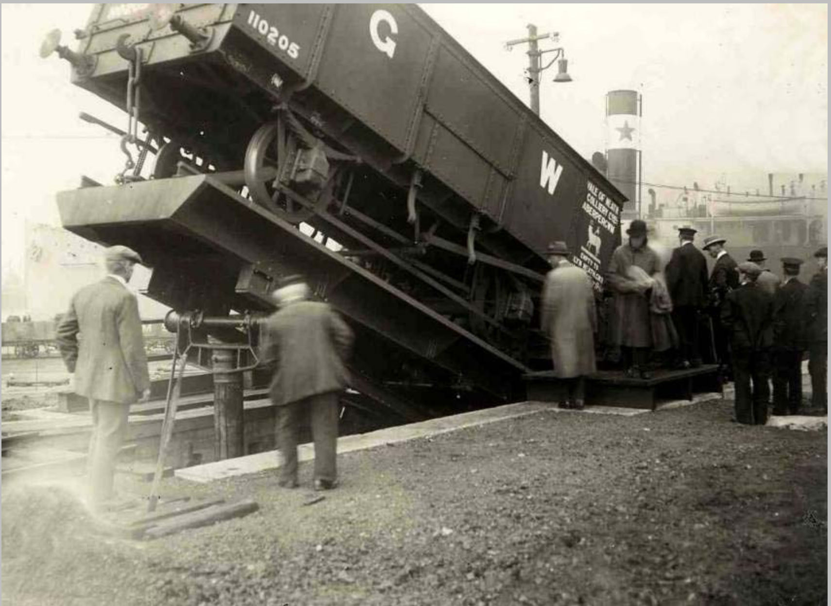
Tipping mechanism at No 3 coal loading conveyor
