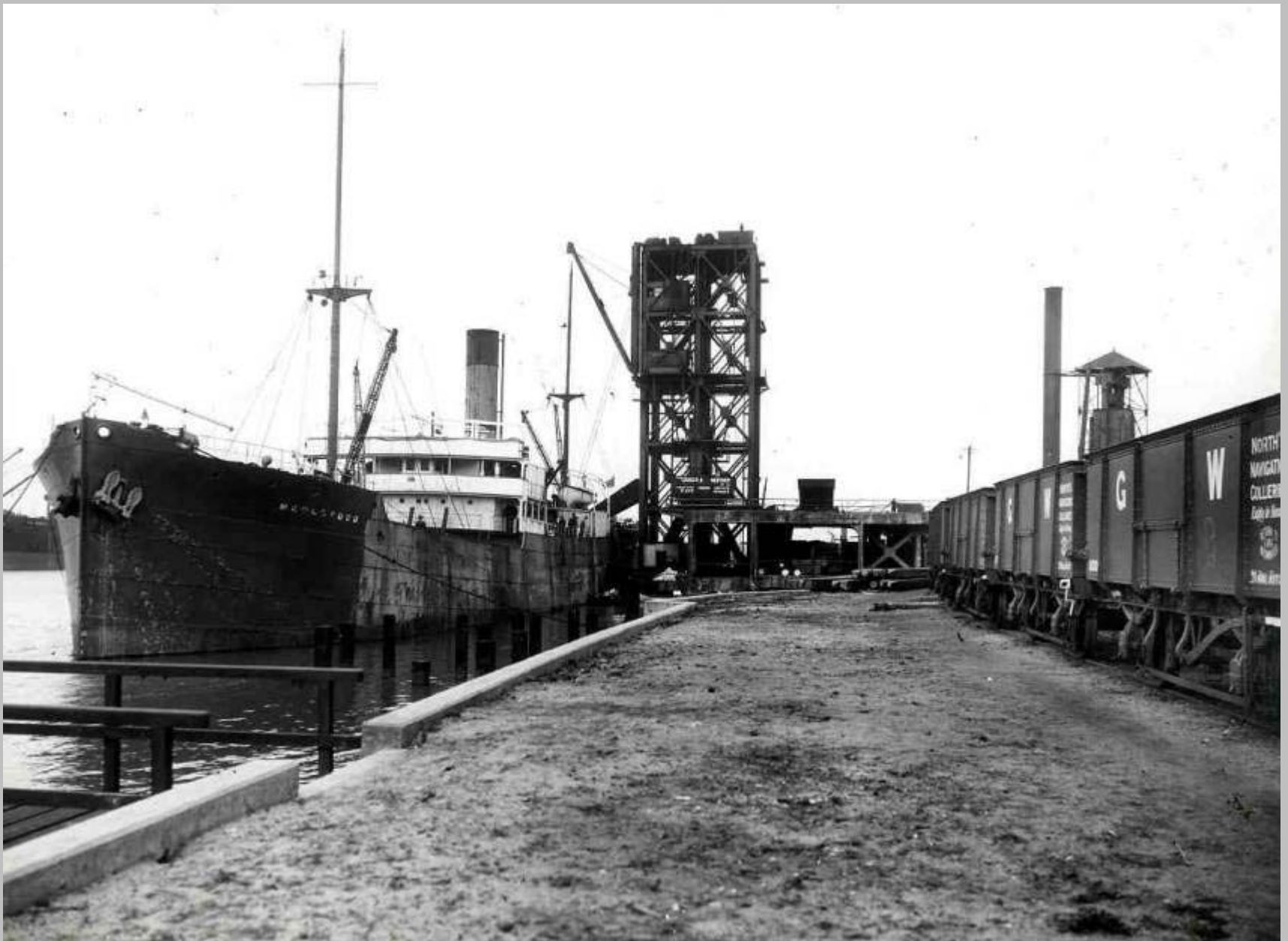
ss 'Maplewood' loading coal in 1928
