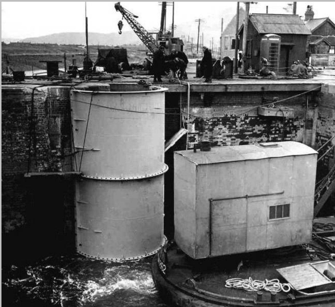
Limpet dam in position at the north outer lock gate 1958
