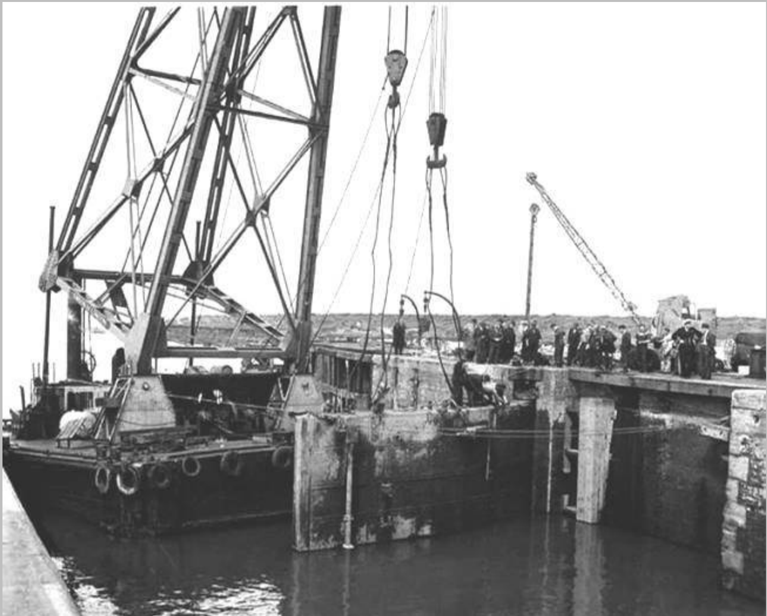
100 ton floating crane taking the weight of north outer lock gate 1958
