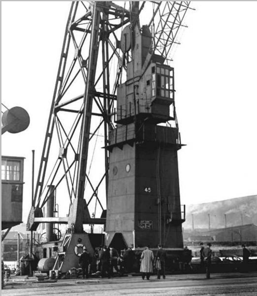
100 ton floating crane landing hydraulic quayside crane on Talbot Wharf in 1946
