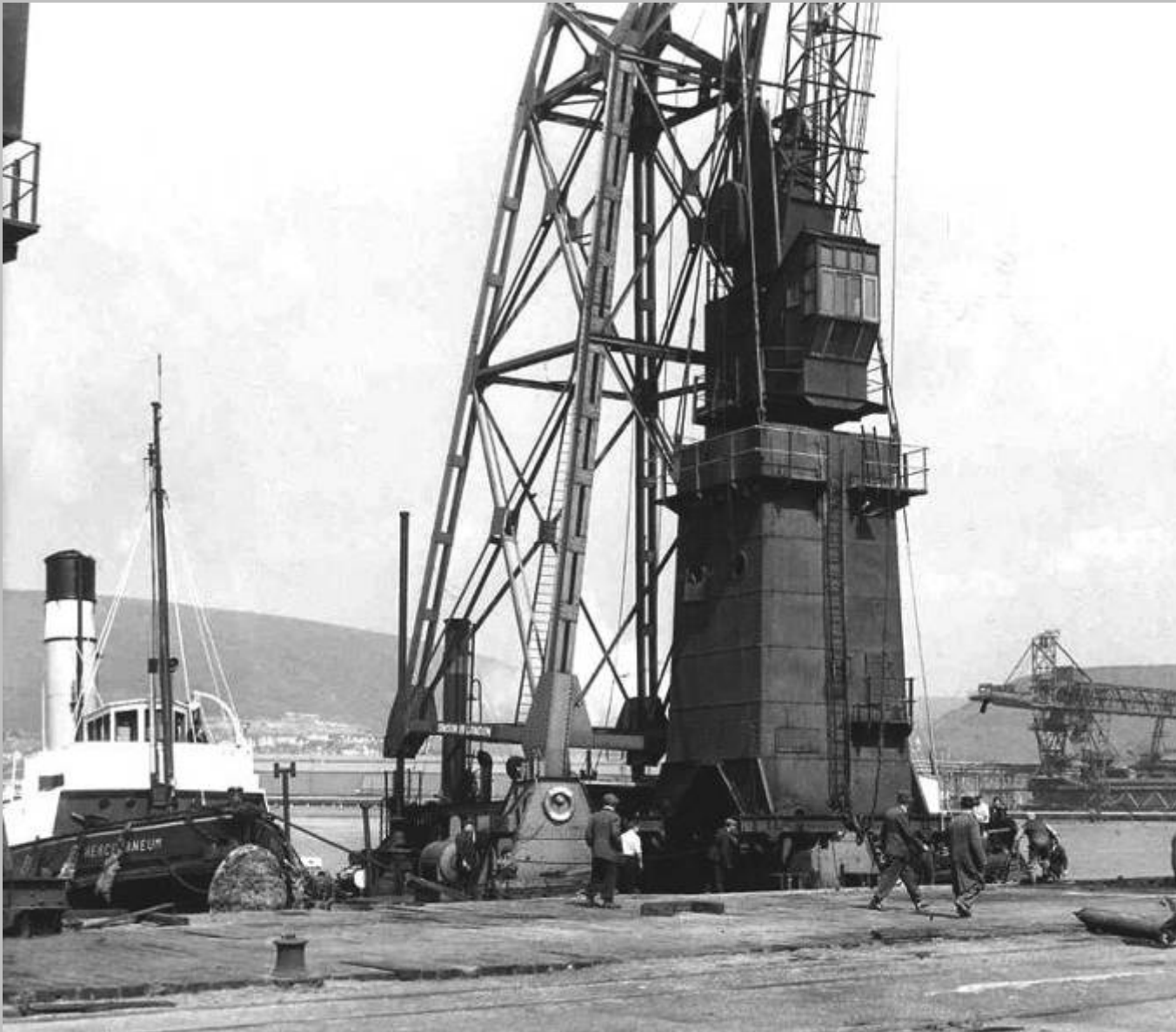
100 ton floating crane landing hydraulic quayside crane on Talbot Wharf – tugs 'Benson' & 'Herculaneum' 1960
