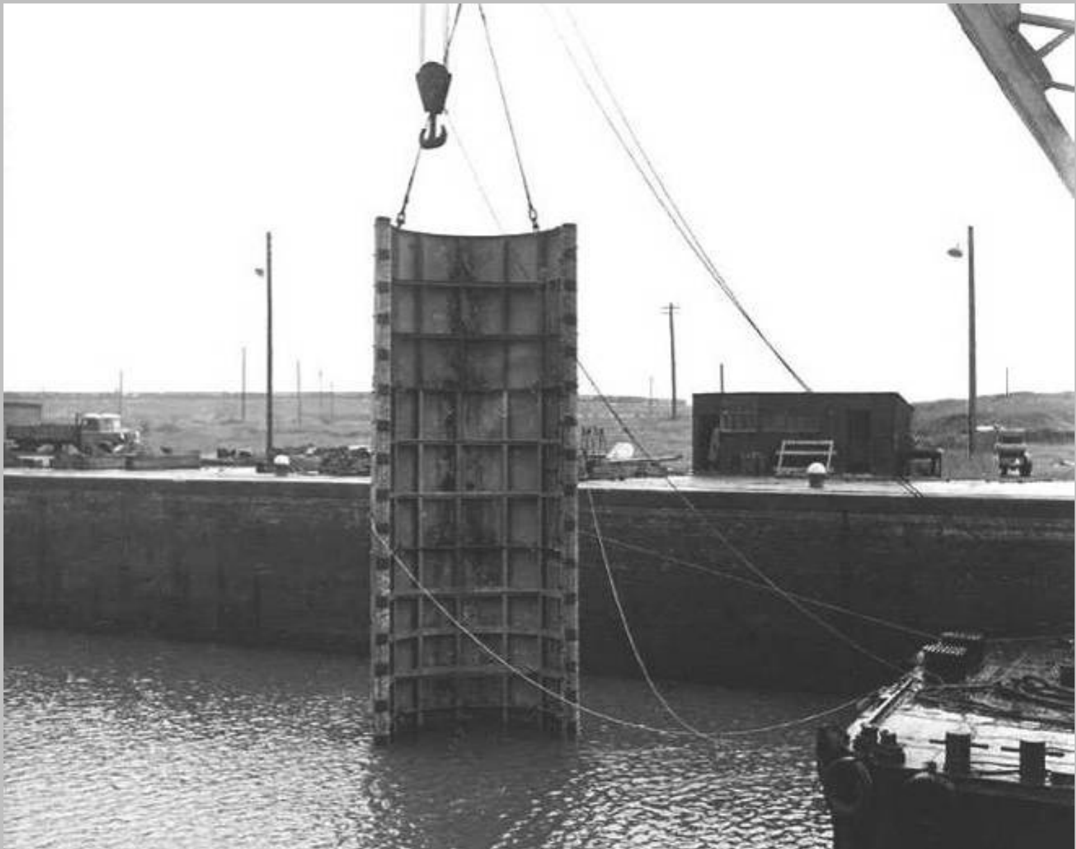
Floating crane carrying limpet dam to north outer lock gate recess 1958
