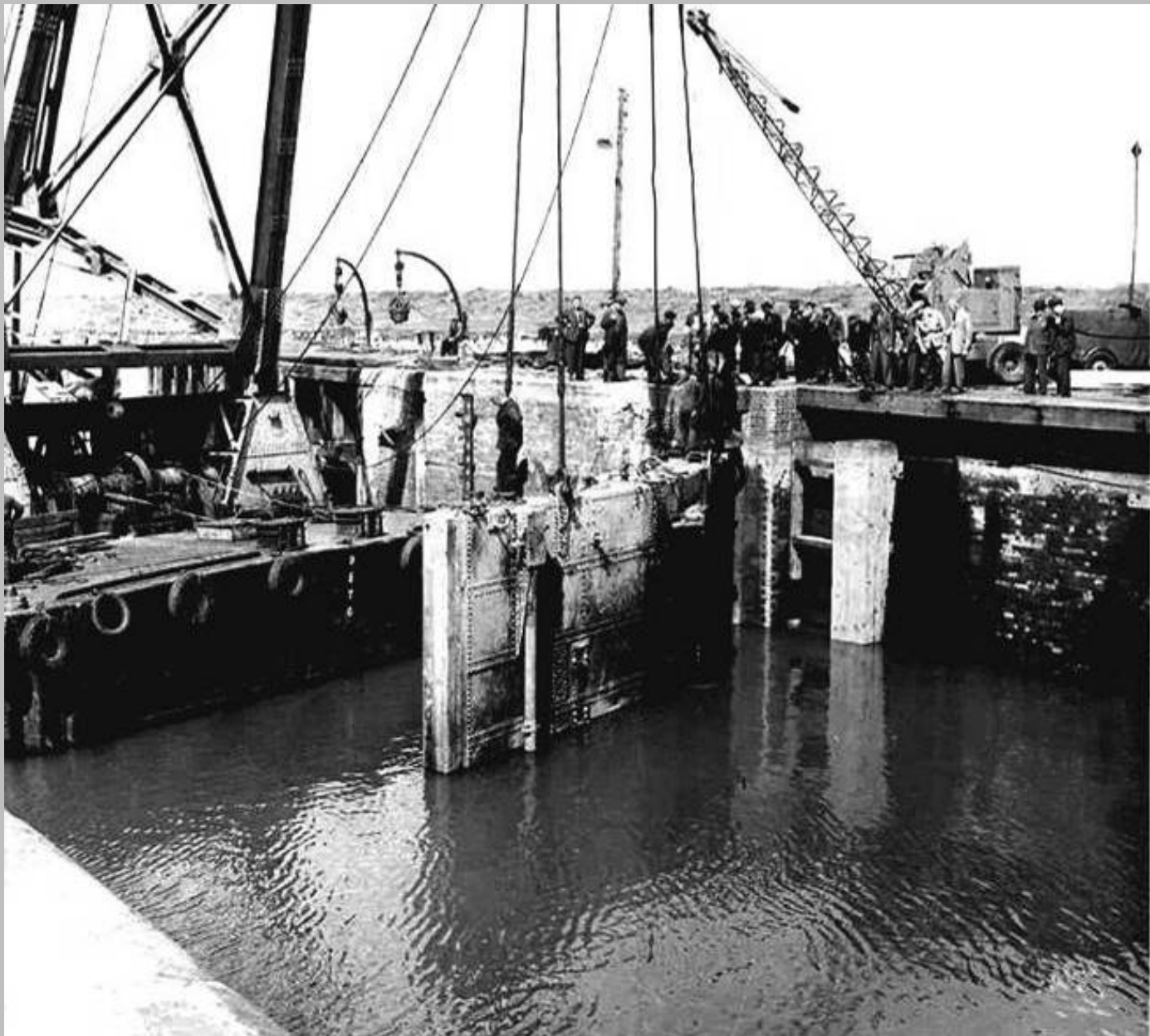
100 ton floating crane preparing to unstep north outer lock gate 1958
