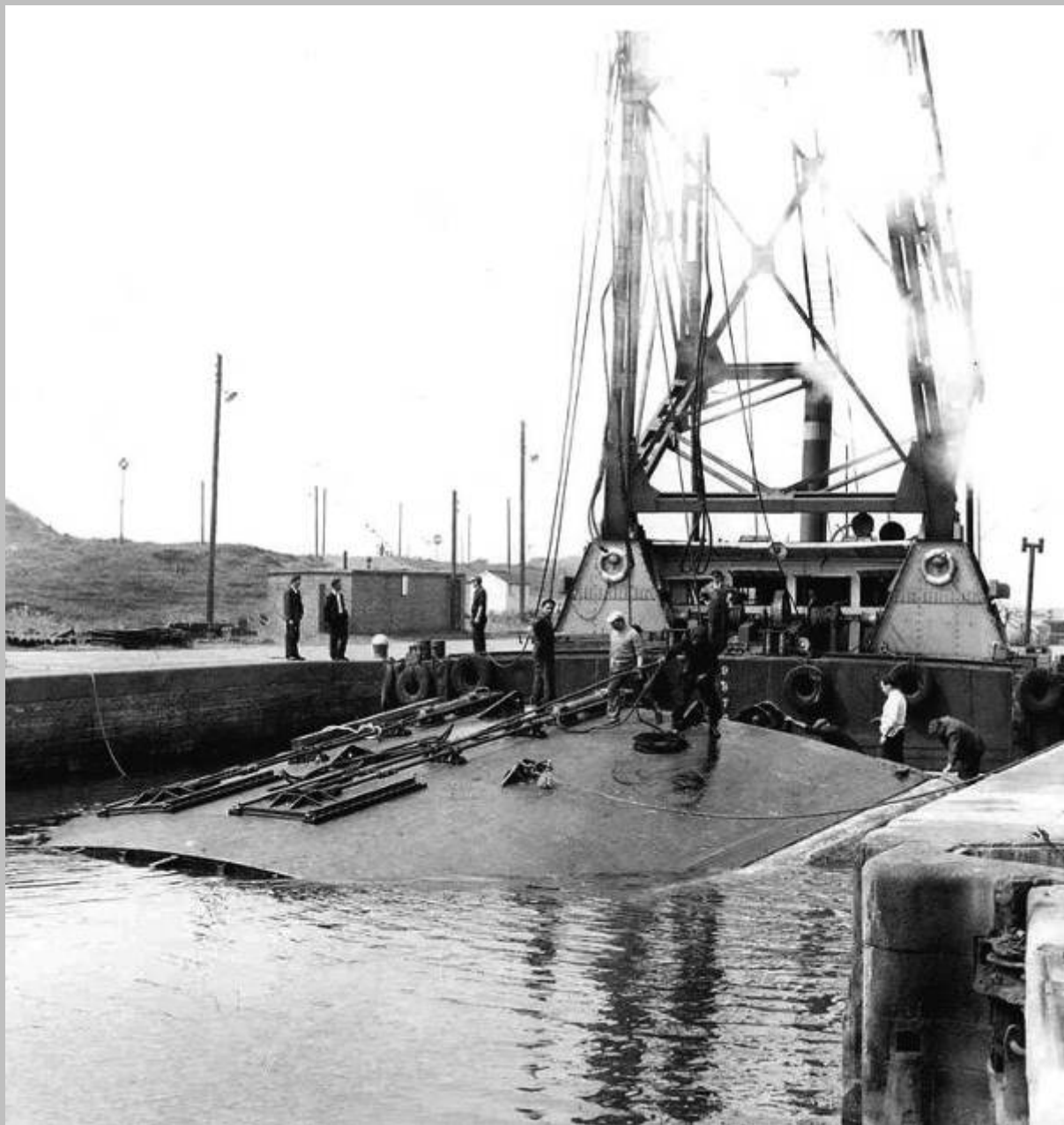
Floating crane in lock with lock gate afloat 1958
