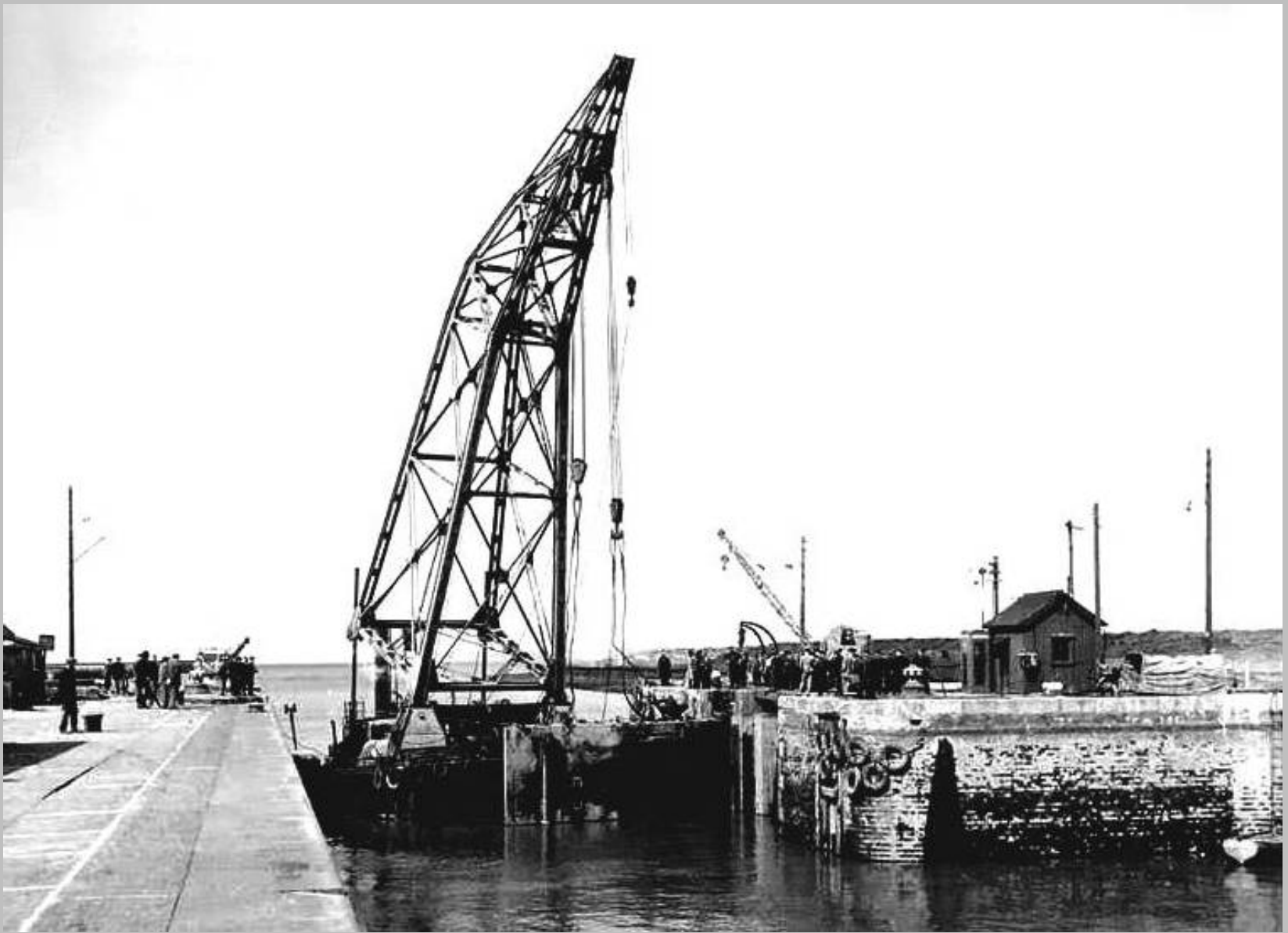
Floating crane entering the locks to unstep the north outer lock gate
