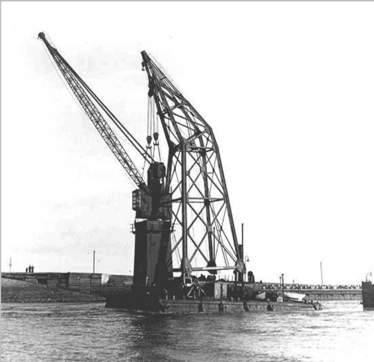
100 ton floating crane carrying hydraulic quayside crane from Barry, approaching Port Talbot lock entrance in 1946.
