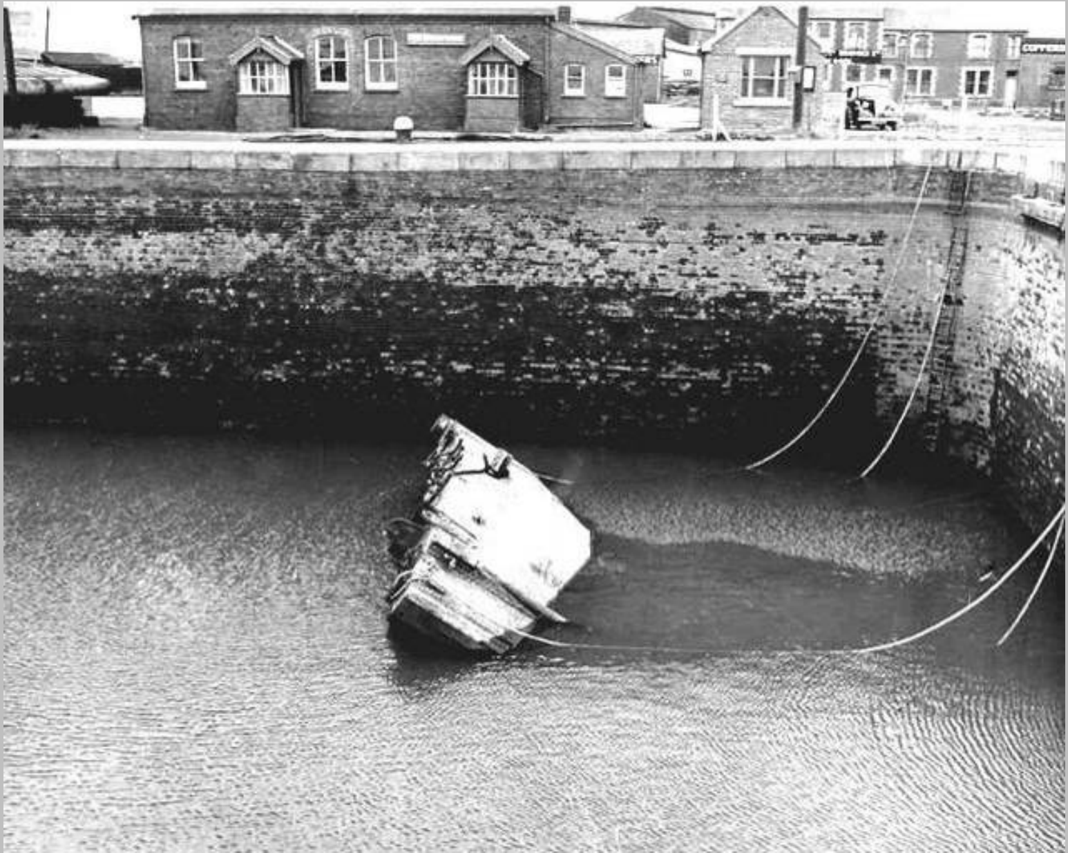
North outer lock gate, semi floating in east end of lock lay by 1958
