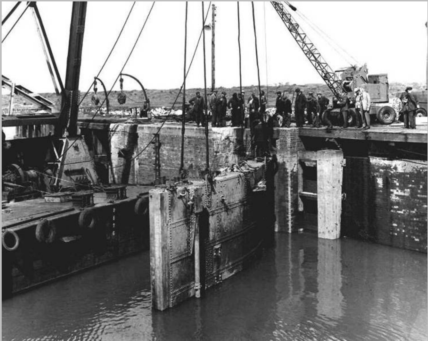
100 ton floating crane preparing to unstep north outer lock gate 1958
