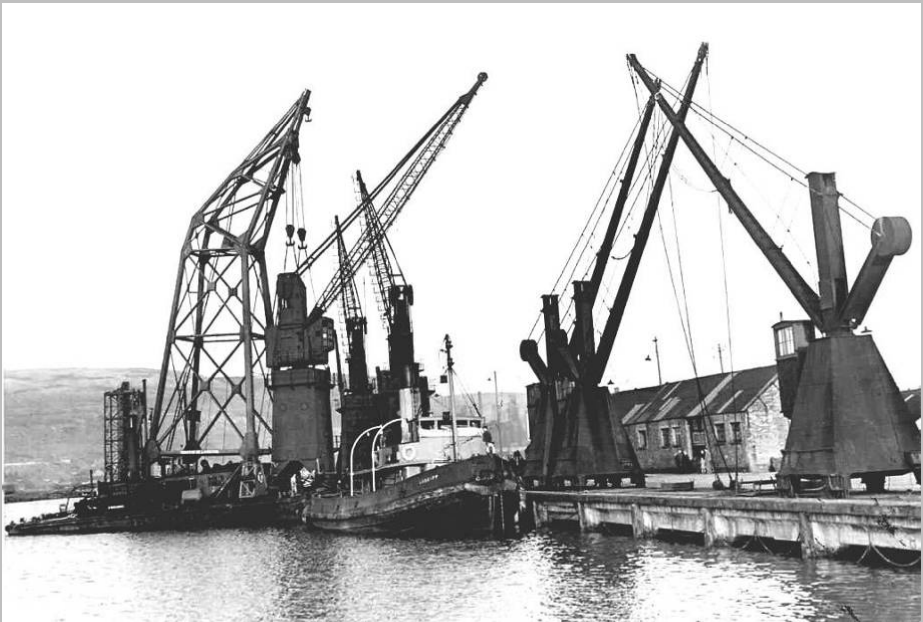
100 ton floating crane landing hydraulic quayside crane on Talbot Wharf in 1946
