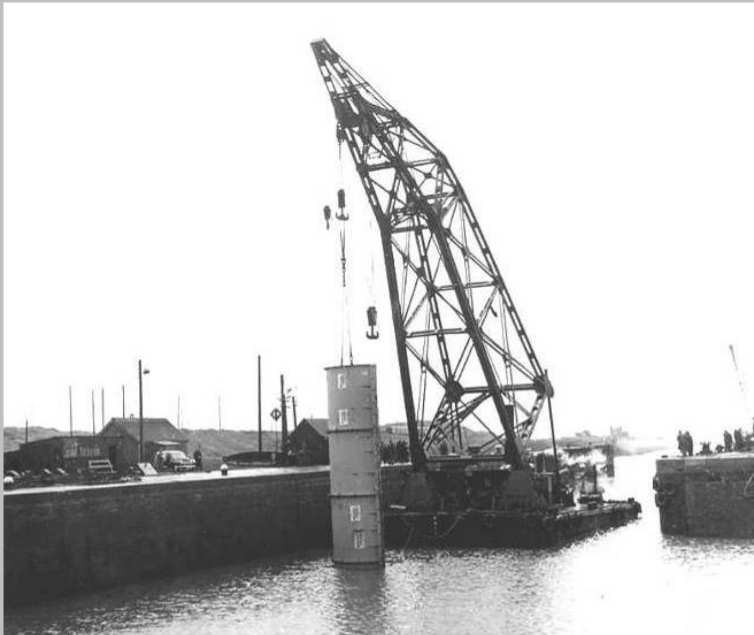
Floating crane carrying limpet dam to north outer lock gate 1958
