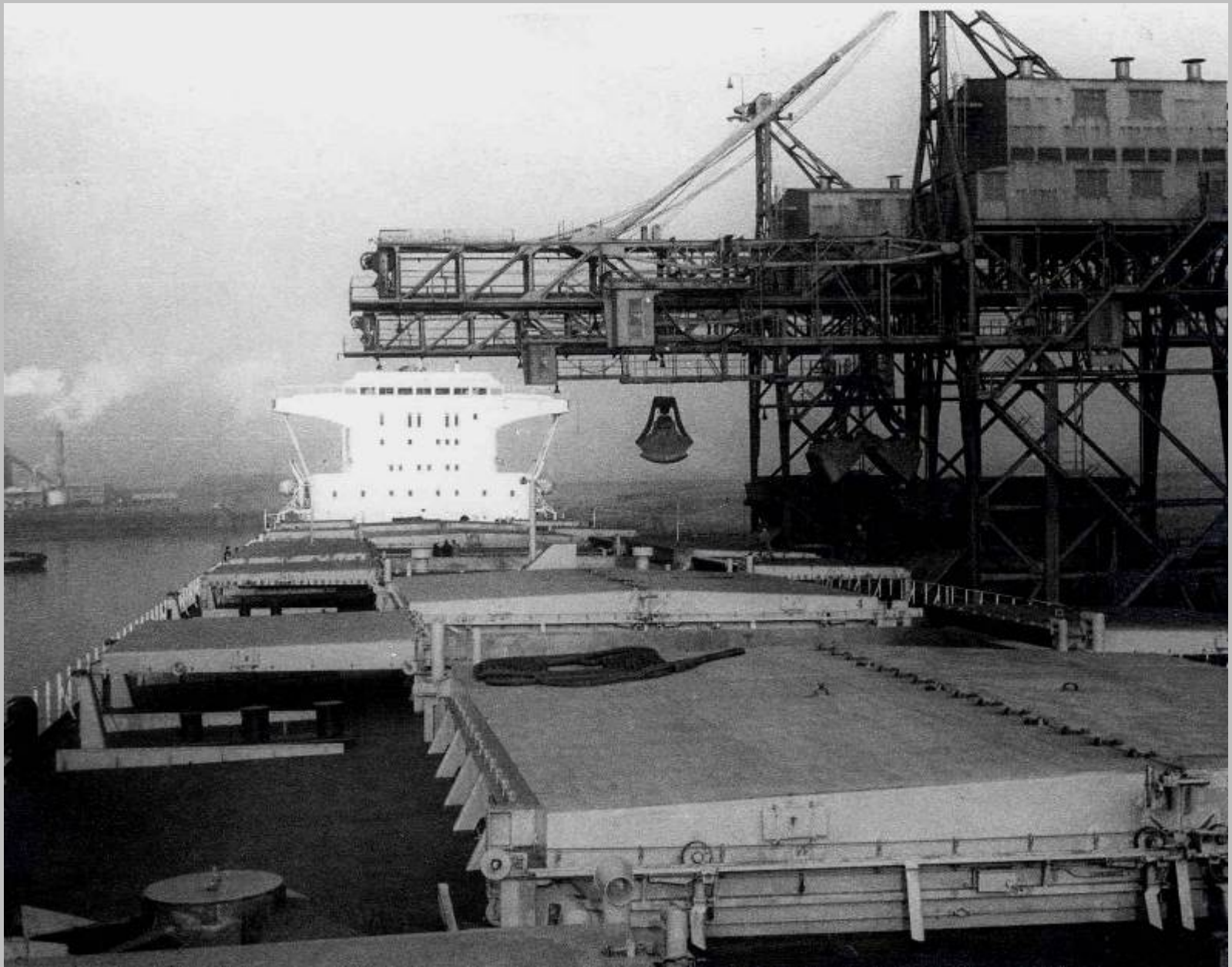
Transporter cranes Margam Wharf
