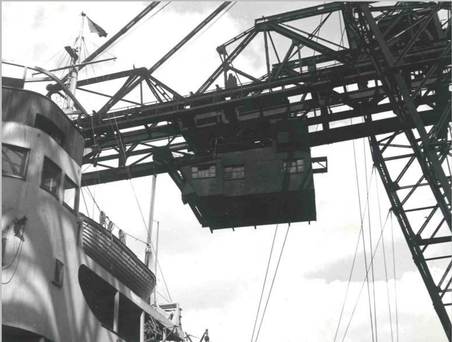
Looking up at the driving cab of the transporter crane
