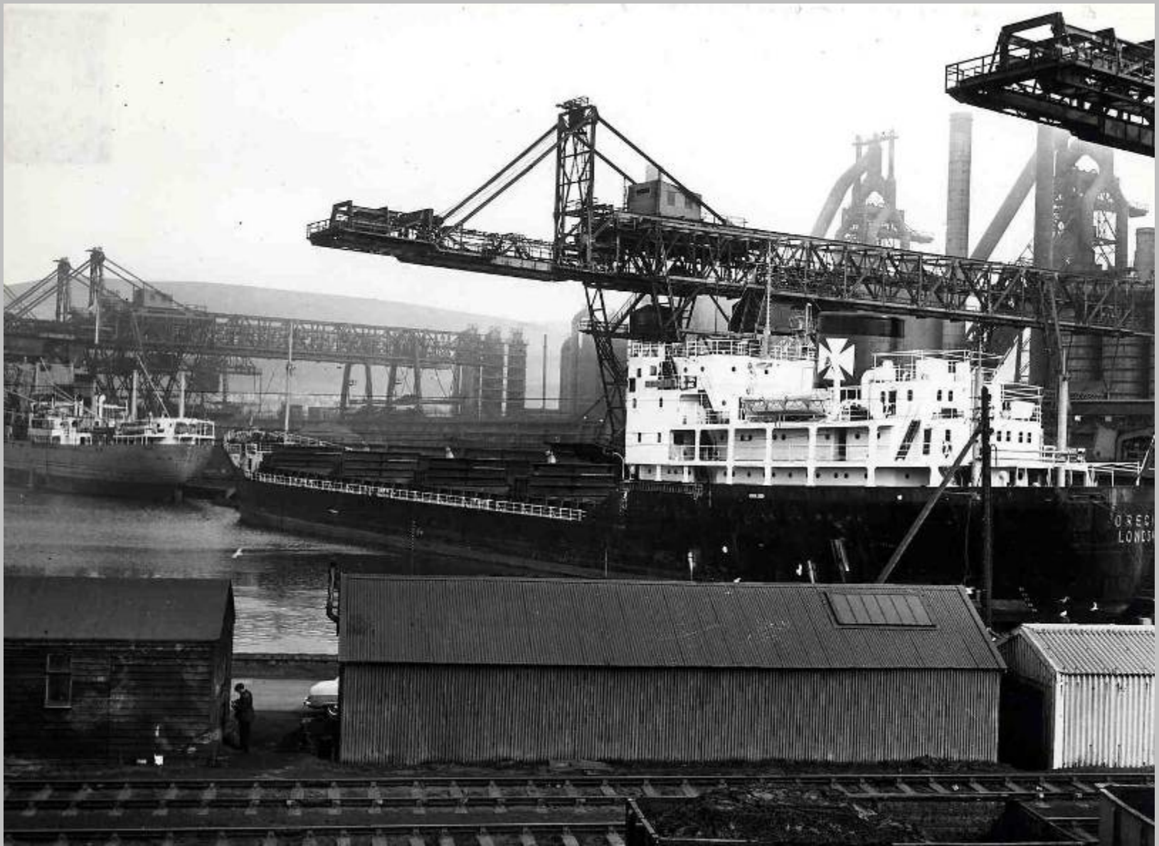
3 Transporter cranes viewed from No. 10 quay
