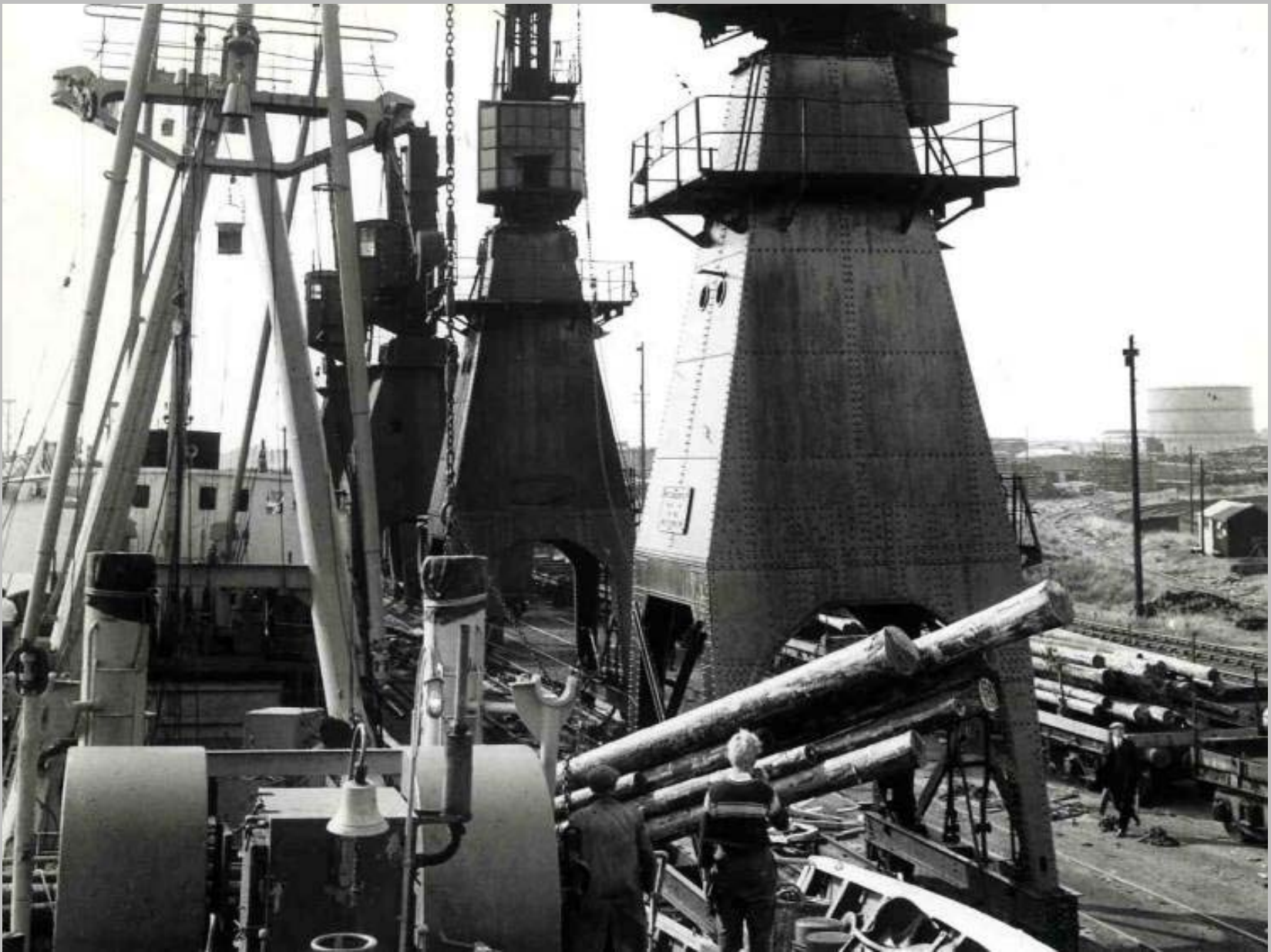
Discharging telegraph poles at Steel Works Wharf
