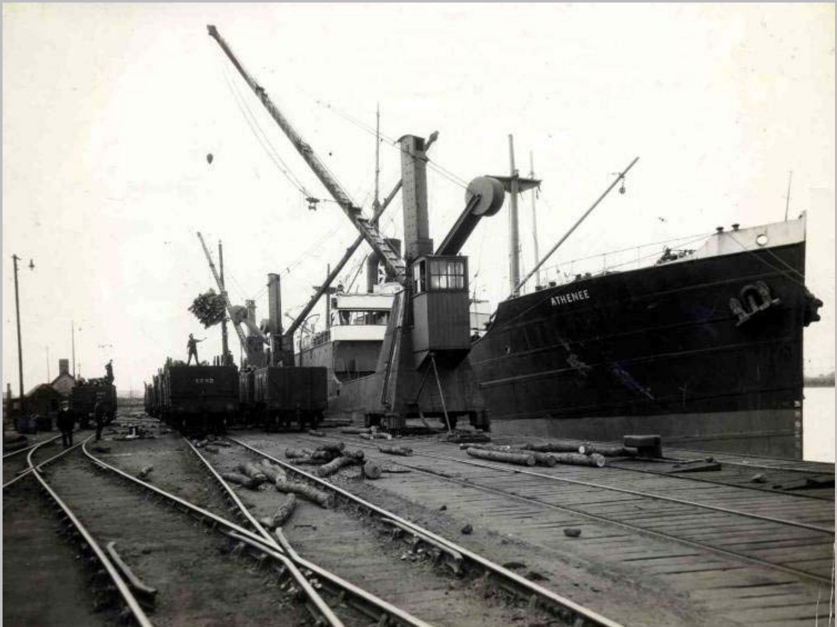
Ss 'Athenee' discharging pitprops at Talbot Wharf in 1927
