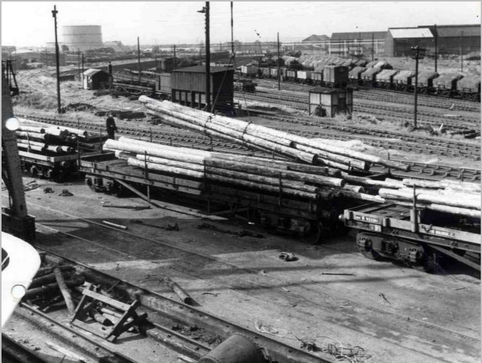
Discharging telegraph poles at Steel Works Wharf
