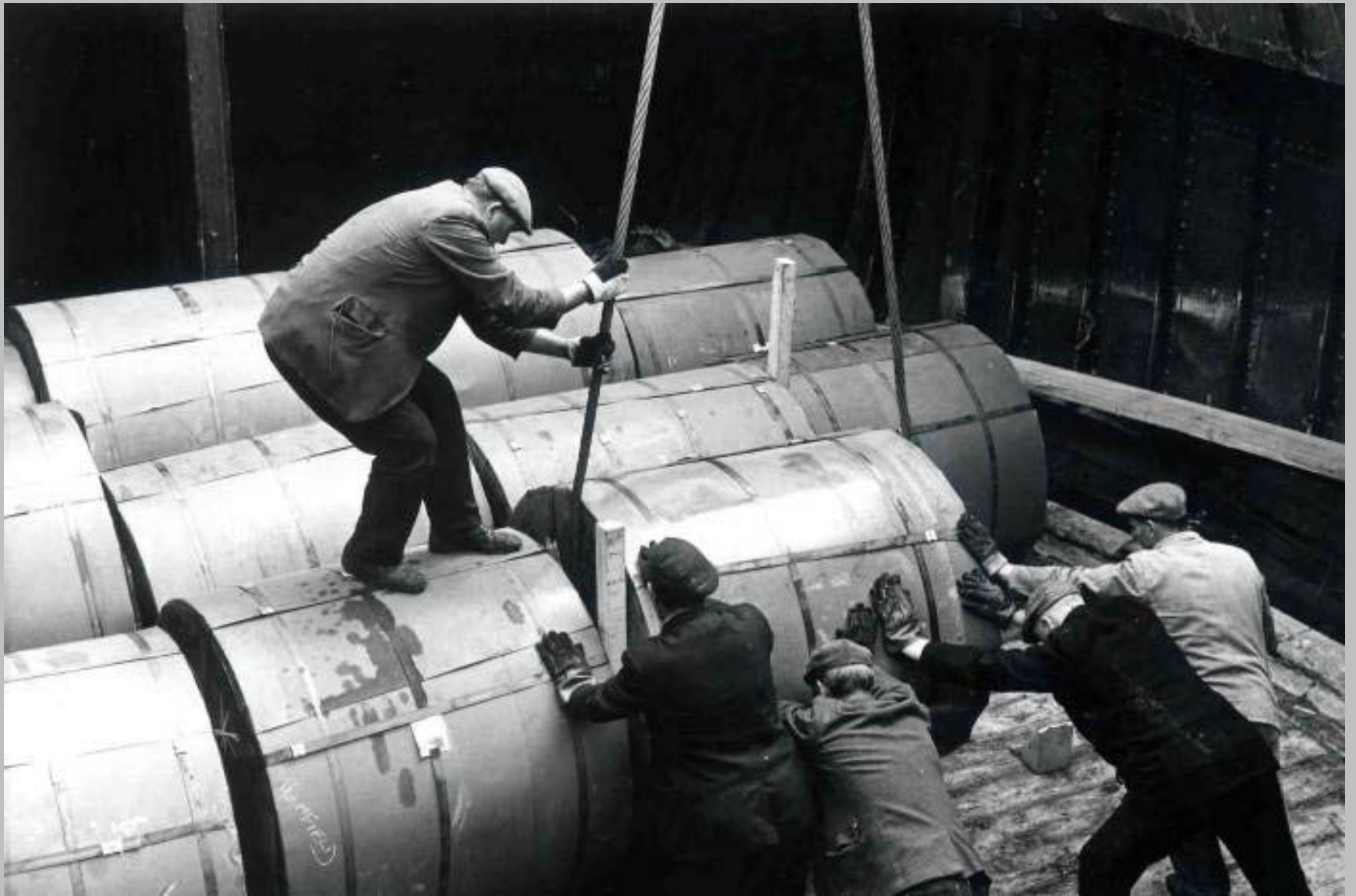
Positioning the coil in order to remove the sling wire
