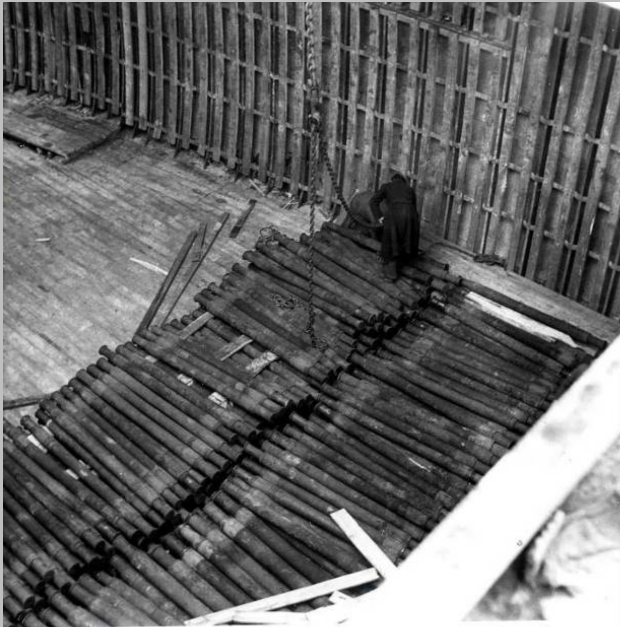
Loading steel billets
