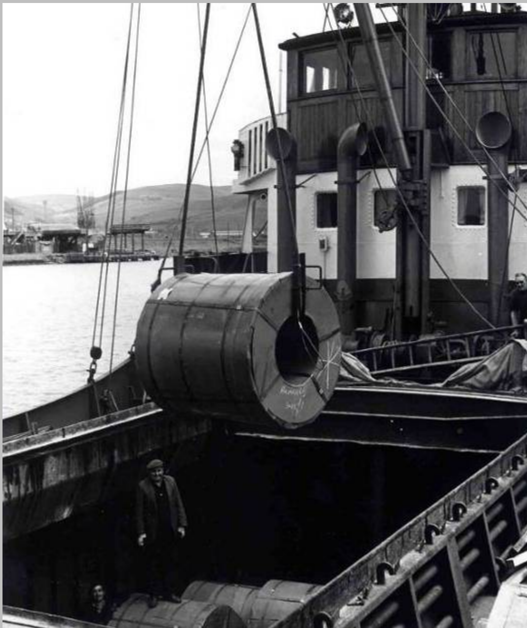
Lowering a steel coil into the hold
