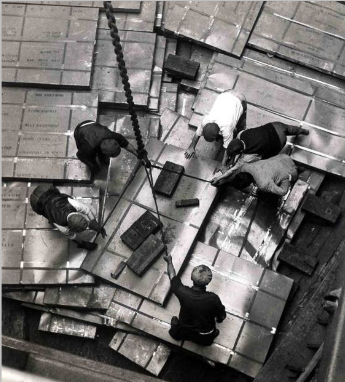
Guiding the bundles of steel sheets into position
