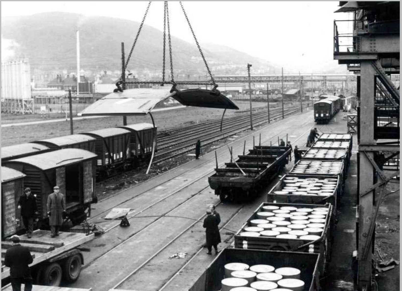
Sling of steel sheets lifted from lorry
